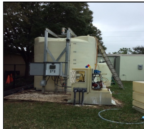
BELOW. The Master Pump Station annual maintenance and cleaning of the 6,500 gallon enhanced alkalinity tank for the chemical injection system used for station and plant process was performed during the reporting month. This was accomplished while keeping the injection system online with a standby tank. Maintenance was performed by Evoqua Water Technologies.
