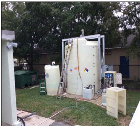
BELOW. The Master Pump Station annual maintenance and cleaning of the 6,500 gallon enhanced alkalinity tank for the chemical injection system used for station and plant process was performed during the reporting month. This was accomplished while keeping the injection system online with a standby tank. Maintenance was performed by Evoqua Water Technologies.
