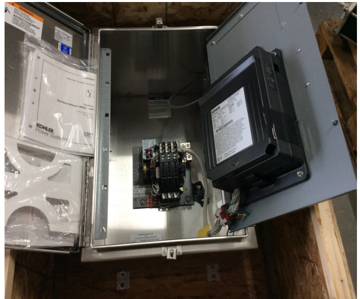
The new ATS for Lift Station 242 was delivered.
