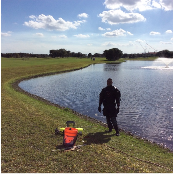
Below: District hired certified diver to plug a backwash pipe that discharges to golf course lake from IQ 518
