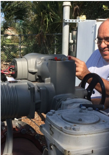
Below: District Electrician/Instrumentation Technician wiring in new spare electric actuator at IQ 516
