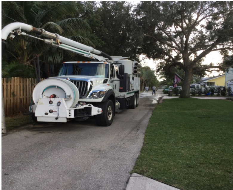
Vac con crew performing street clean up after road side force main repair
