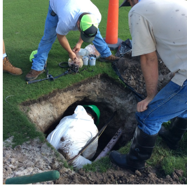
District Construction crew performed repair to failed 45 degree pipe bend after pipe plugged in lake and strainer system isolated
