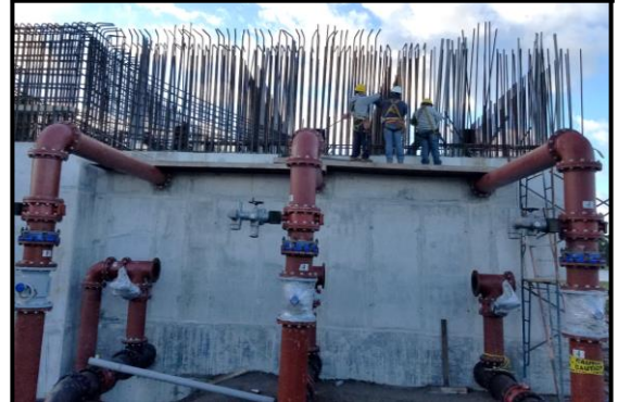
Installation of Filter Influent and Effluent Piping
