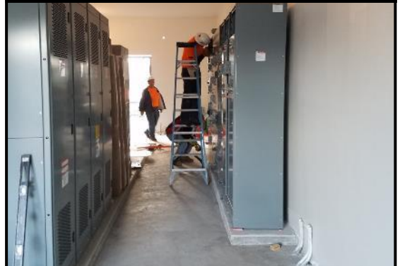
Installation of Equipment in Filter Electrical Building
