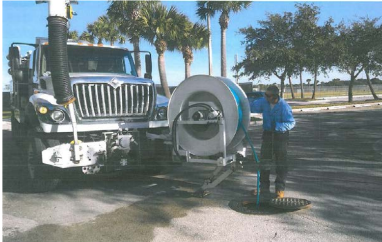
Vaccon crew performing annual gravity main line cleaning on Roger Dean Stadium interior complex.
