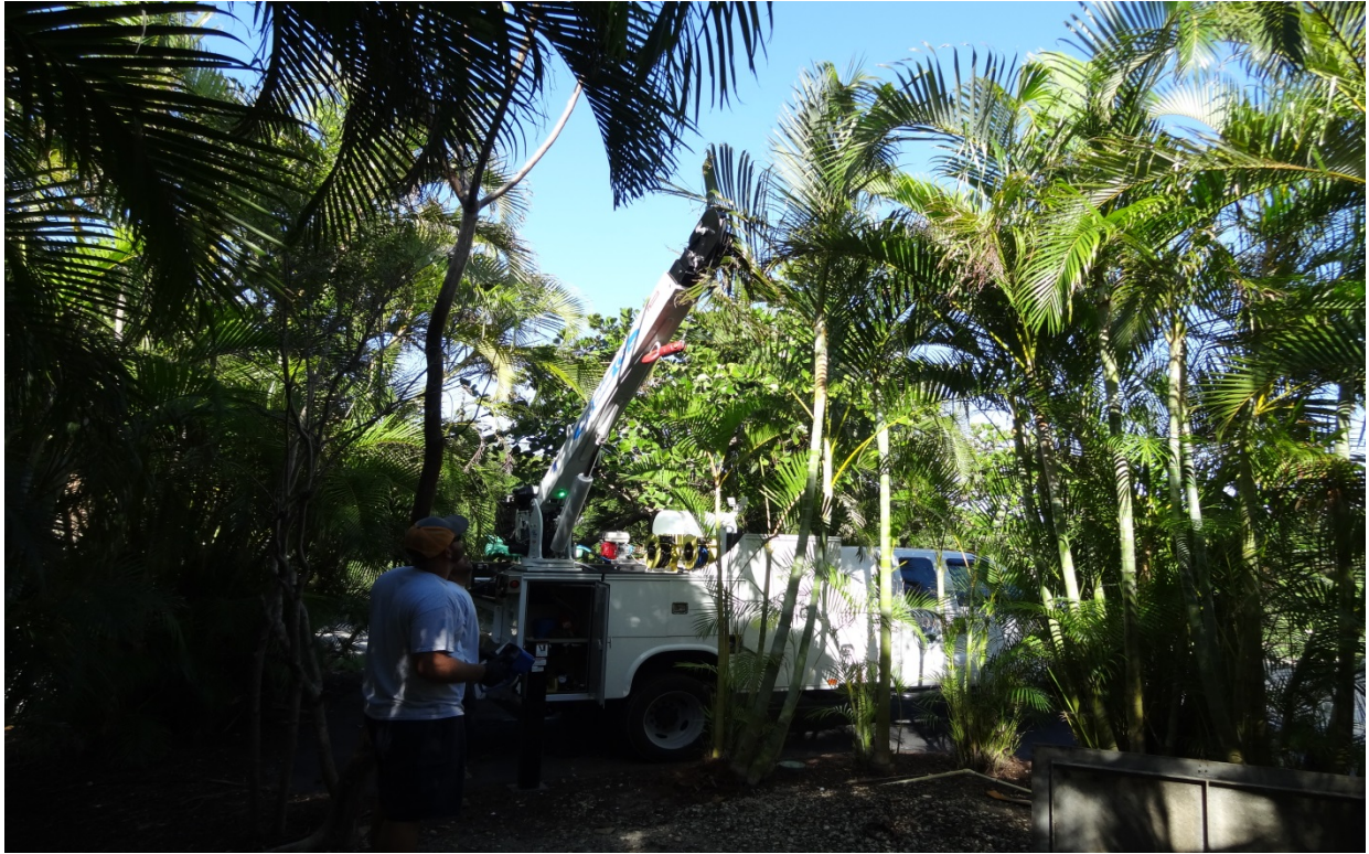
Collections crews preparing to perform inspection, evaluation and preventative maintenance on a lift station.
