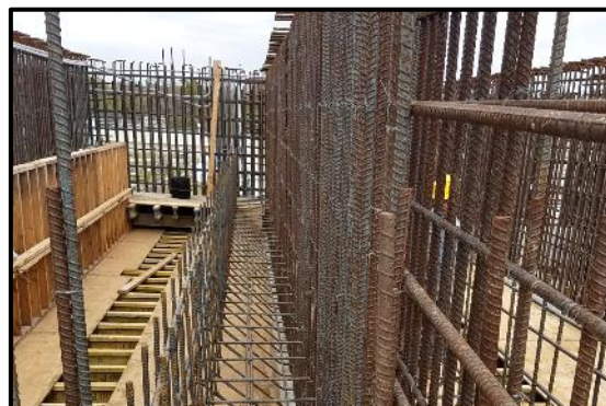
Installation of Steel Reinforcement in West Filter Cell
