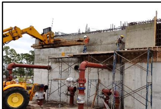
Removal of Formwork at Deep Bed Filter Northeastern Upper Wall Segment
