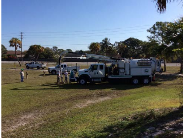
Vaccon #15 assisting the District Construction crew on the plant site to investigate work for future corrective work order
