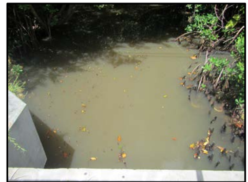
Observed turbidity plume at the Caloosahatchee culvert on July 20.
