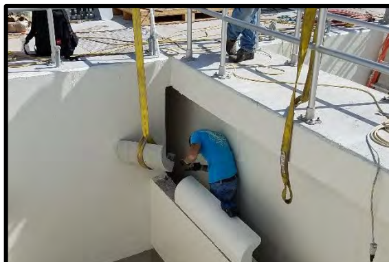
Installation of DBF Cell Weir Blocks
