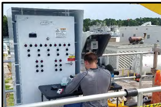
Wiring of DBF Local Panels
