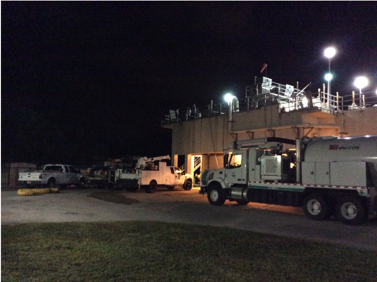
Scheduled night work at Headworks (District) and also for Deep Bed Filters work (Kirlin) at Filter Pump Station #1
