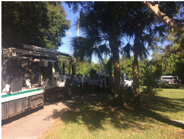
Vac con and Collections crew cleaning lift station #161 for confined space entry inspection
