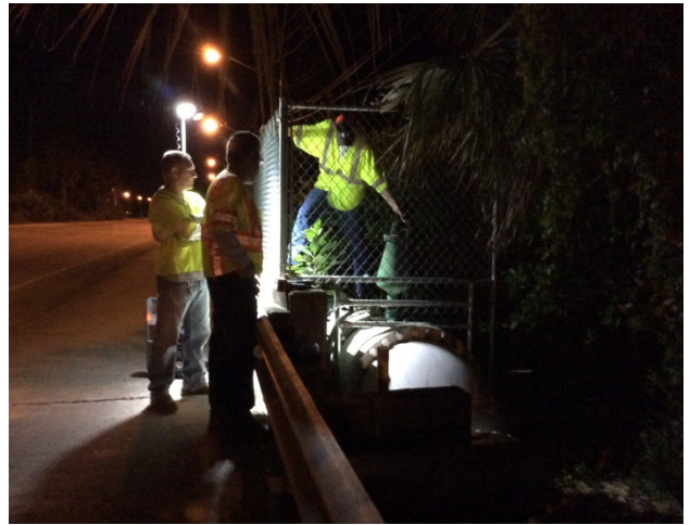
Annual valve exercising and air release valve repairs were performed in field during the collection system shutdown.
