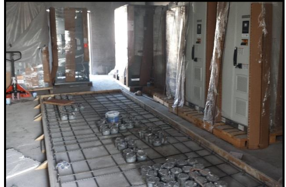
Installation of Housekeeping Pads and Equipment in Filter Electrical Building
