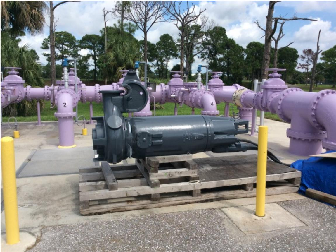
*Plant Master Reuse pump station Factory refurbished 335 HP submersible pump ready for installation*
