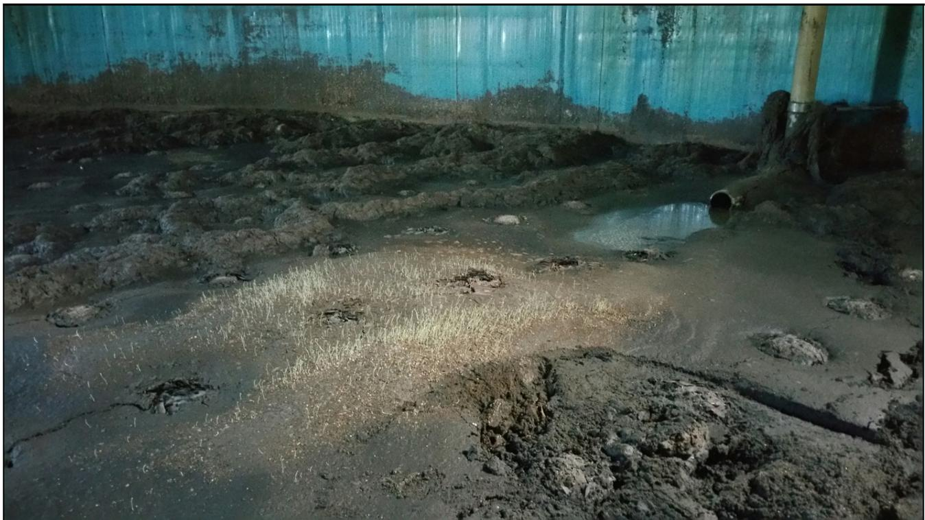
**BELOW.** Toward the end of the project, the diffusers had become exposed and the level of sand and sludge was directed to the lowest point of the tank.
