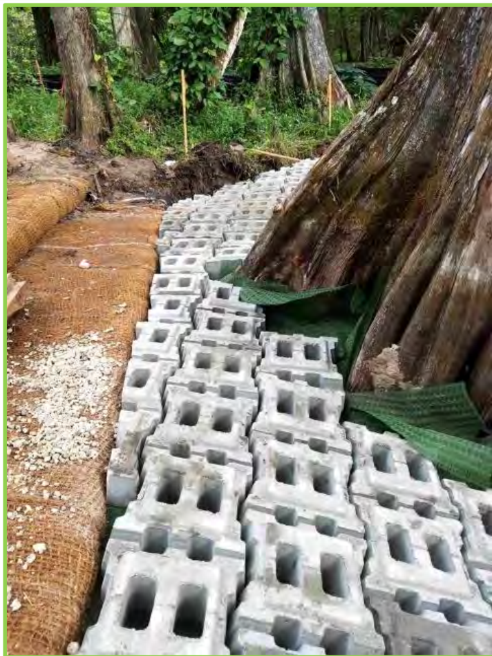
VRSS construction and articulated block placement
