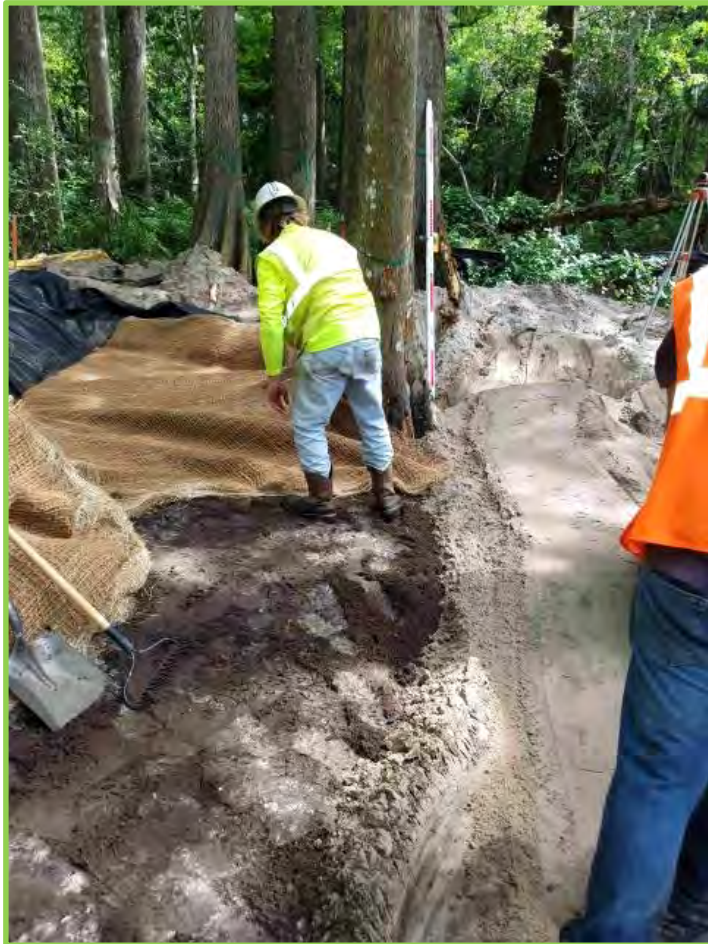
Installing blankets in Alluvial area for the VRSS
