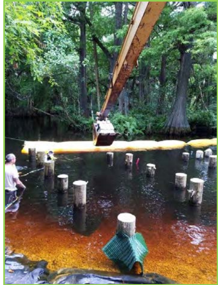
Placing bedding stone to protect slopes from erosion
