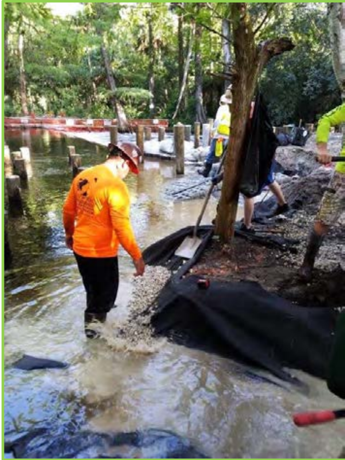
Placing bedding stone to protect slopes from erosion
