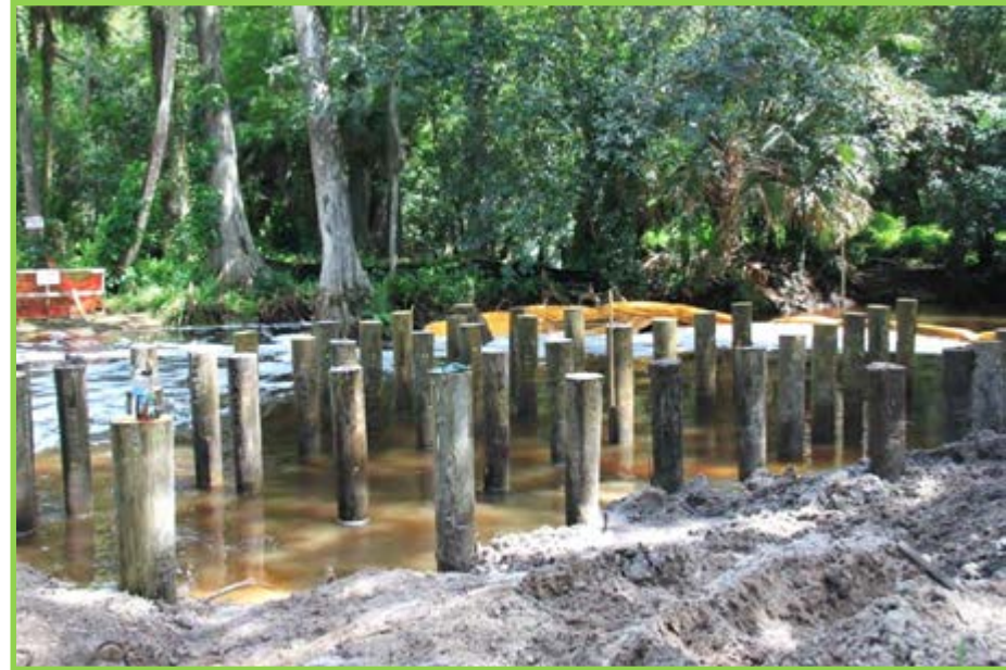
Pilings for the portage and benches on East side of Masten Dam
