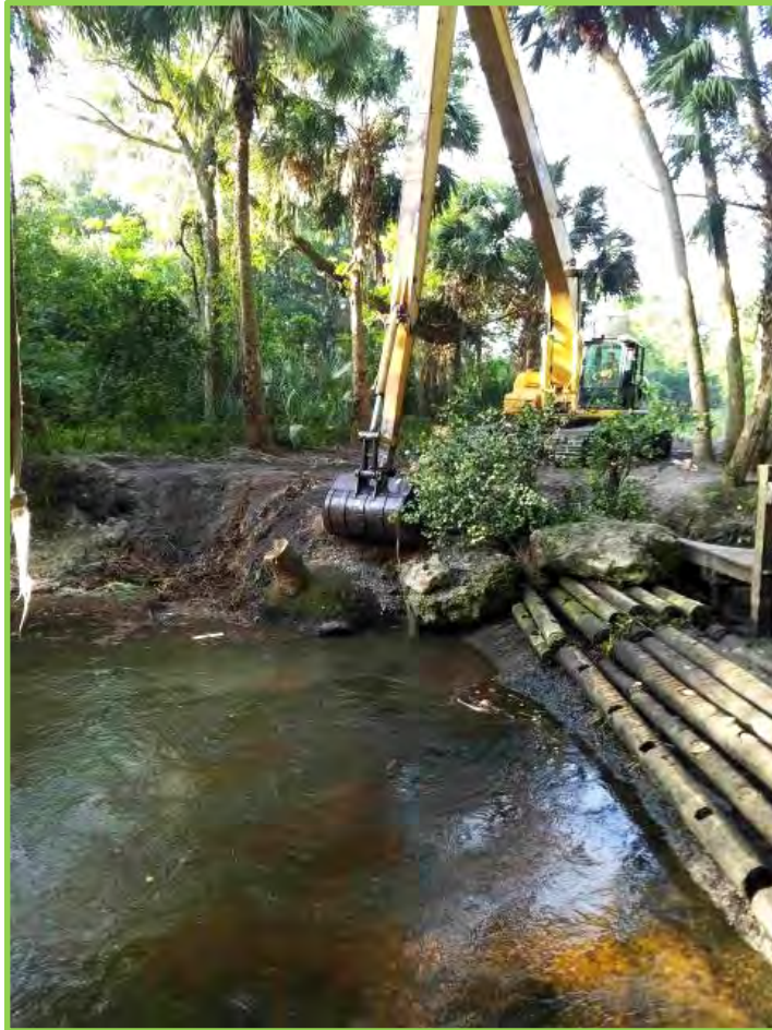
Clearing and demolition on East side of the Lainhart Dam
