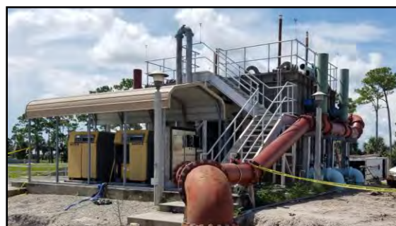
Modification of the Synthetic Media Filter Piping
