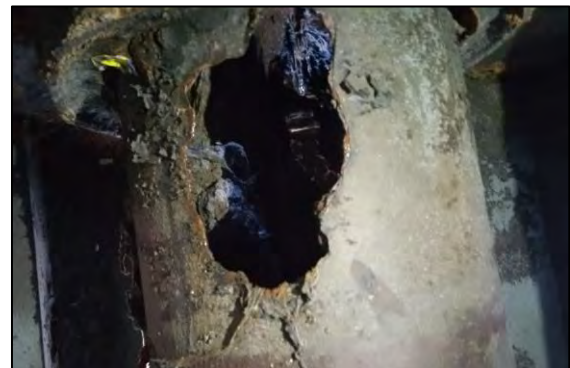
Clarifier No. 3 Column Condition
