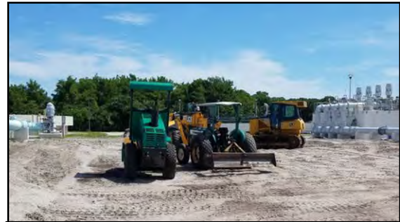
Continuation of Final Site Grading
