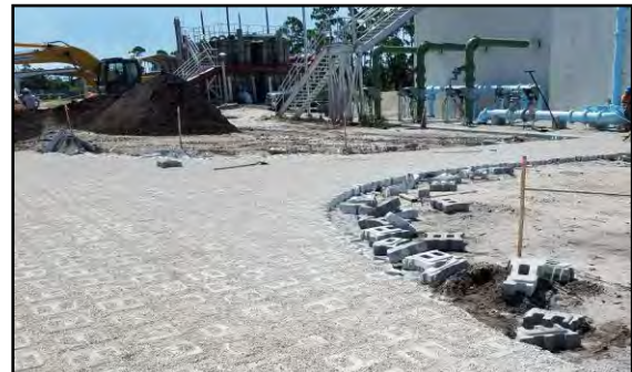
Installation of New Paver Roadway
