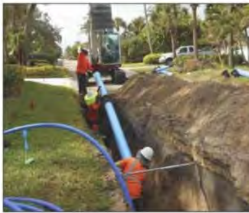
A new water main pipe being installed.
