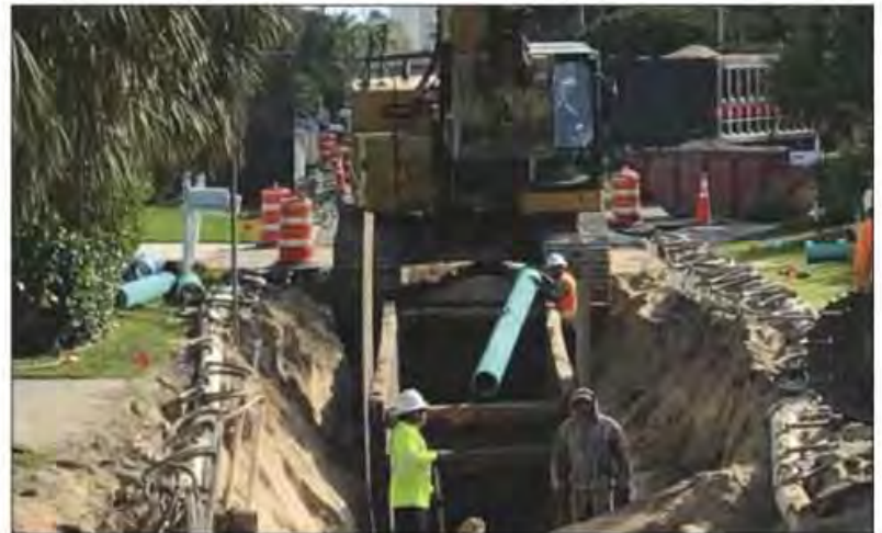
Heavy equipment is used for the project during installation of the gravity sewer.
