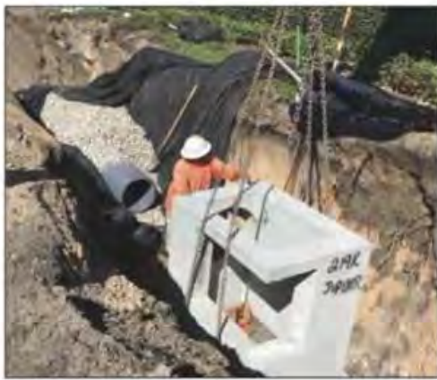
Installing the exfiltration trenches.
