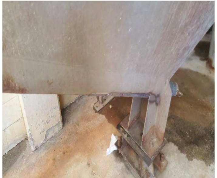
Grit Classifier Unit - Repair Plates
