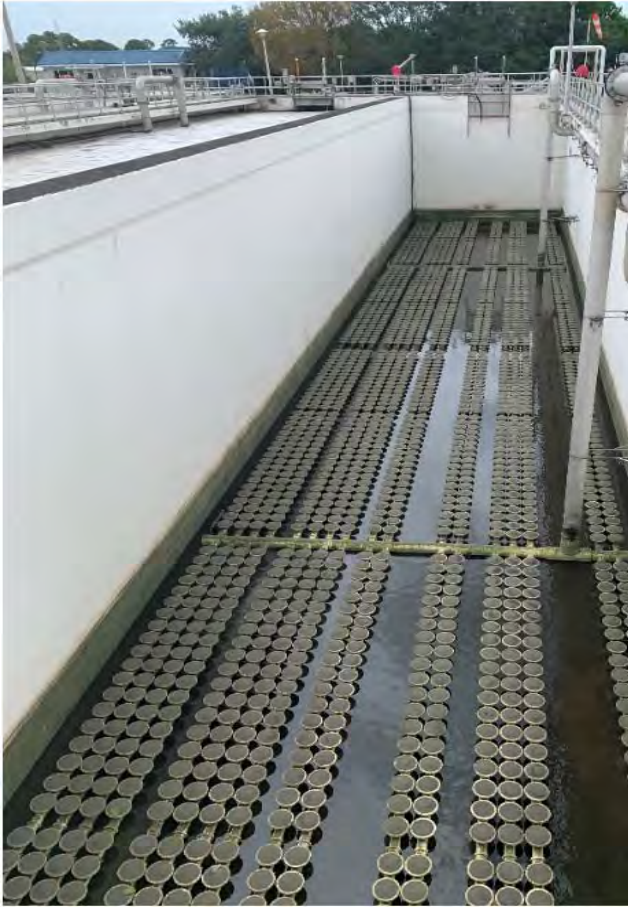
Aeration Basin No. 1 – Fine Bubble Diffusers and Piping
