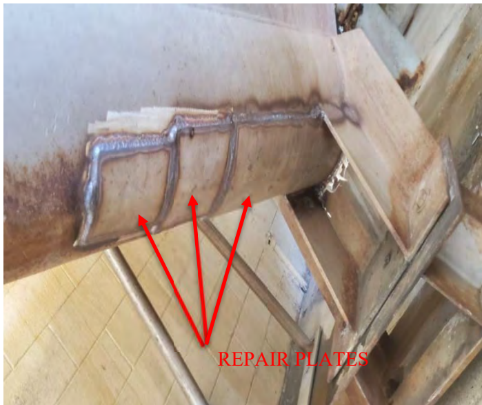
Grit Classifier Unit - Repair Plates
