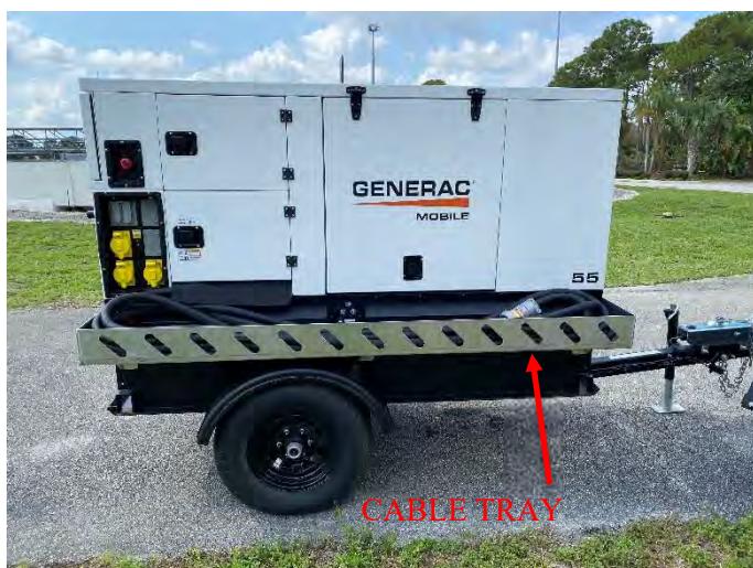
Towable Emergency/Standby Generator Unit – Cable Trays
