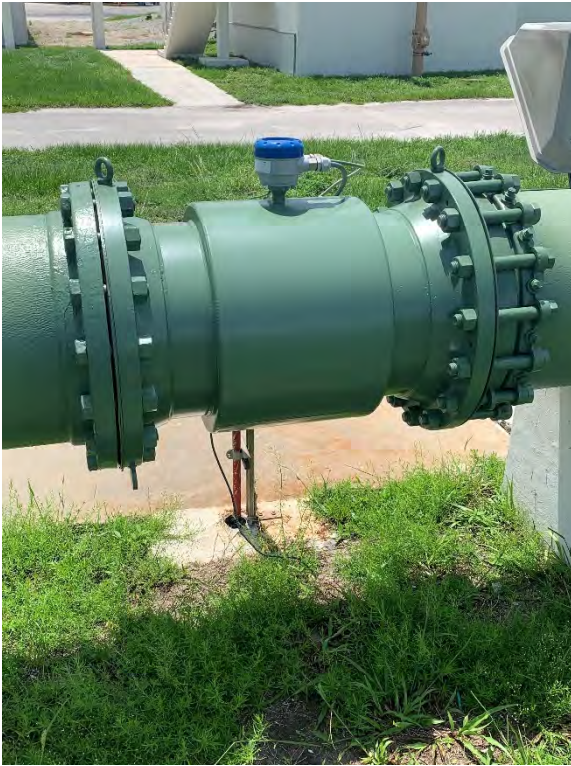
Filter Pump Station No. 2 – Inline Flow Meter
