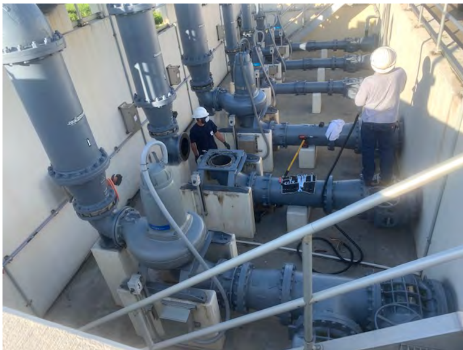
EQ Pump Station – Pump Removal
