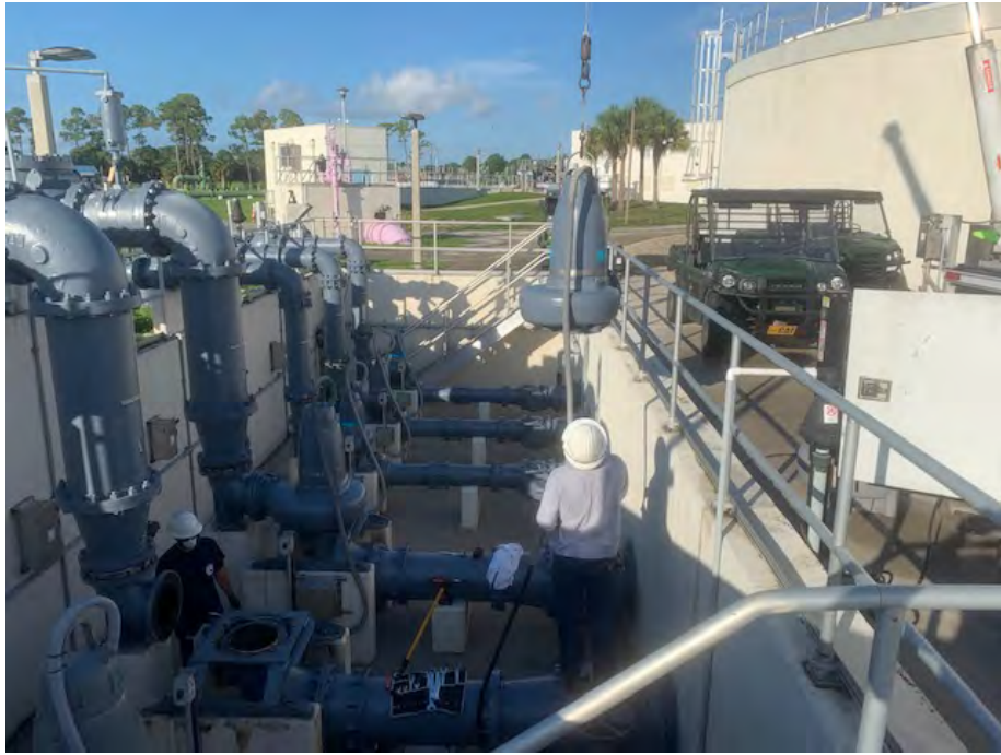
EQ Pump Station – Pump Removal
