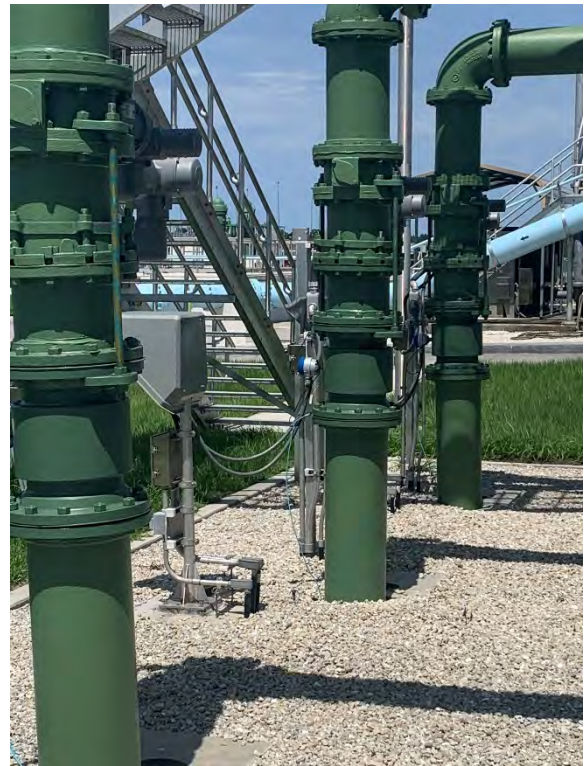
Deep Bed Filters – Inline Flow Meters/Piping
