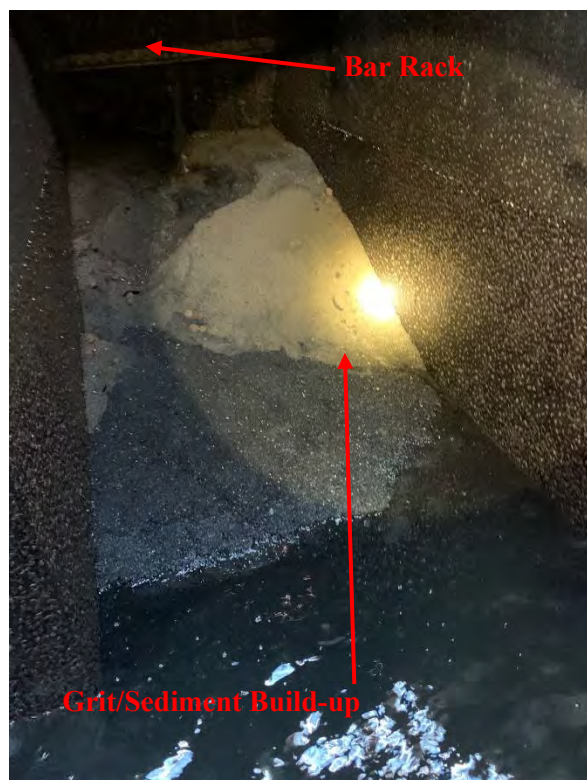
Injection Well Bar Rack Structure – Pre-Clean-Out Photos
