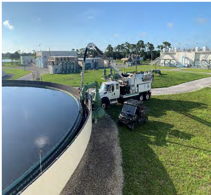
Clarifier Effluent Box Rack – Clean-Out Photo Nos. 1 and 2
