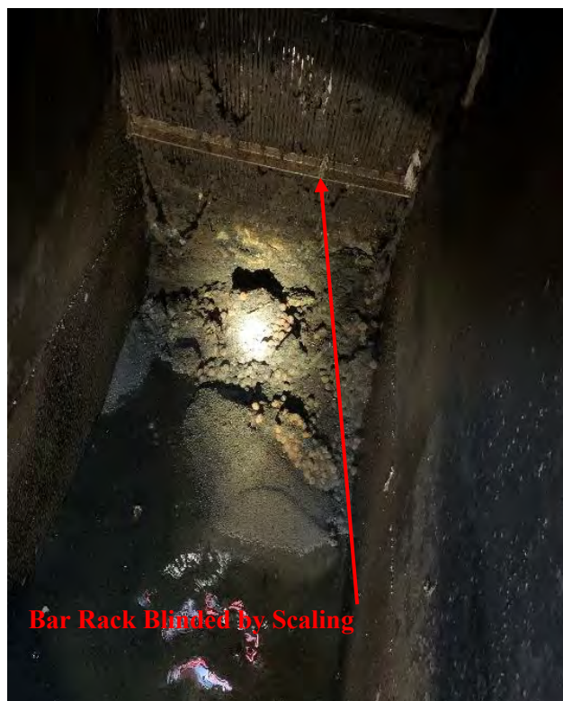
Injection Well Bar Rack Structure – Pre-Clean-Out Photos
