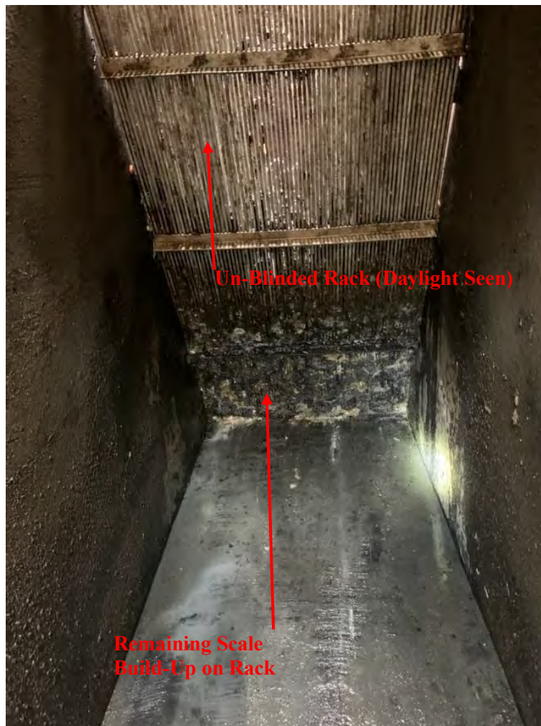
Injection Well Bar Rack Structure – Post-Clean-Out Photo
