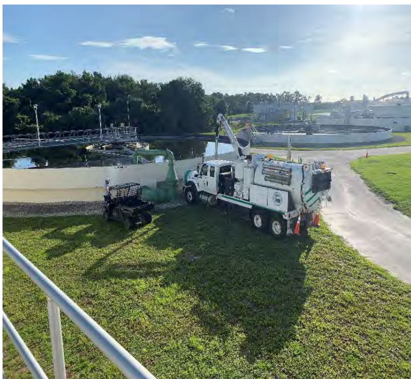
Clarifier Effluent Box Rack – Clean-Out Photo No. 3
