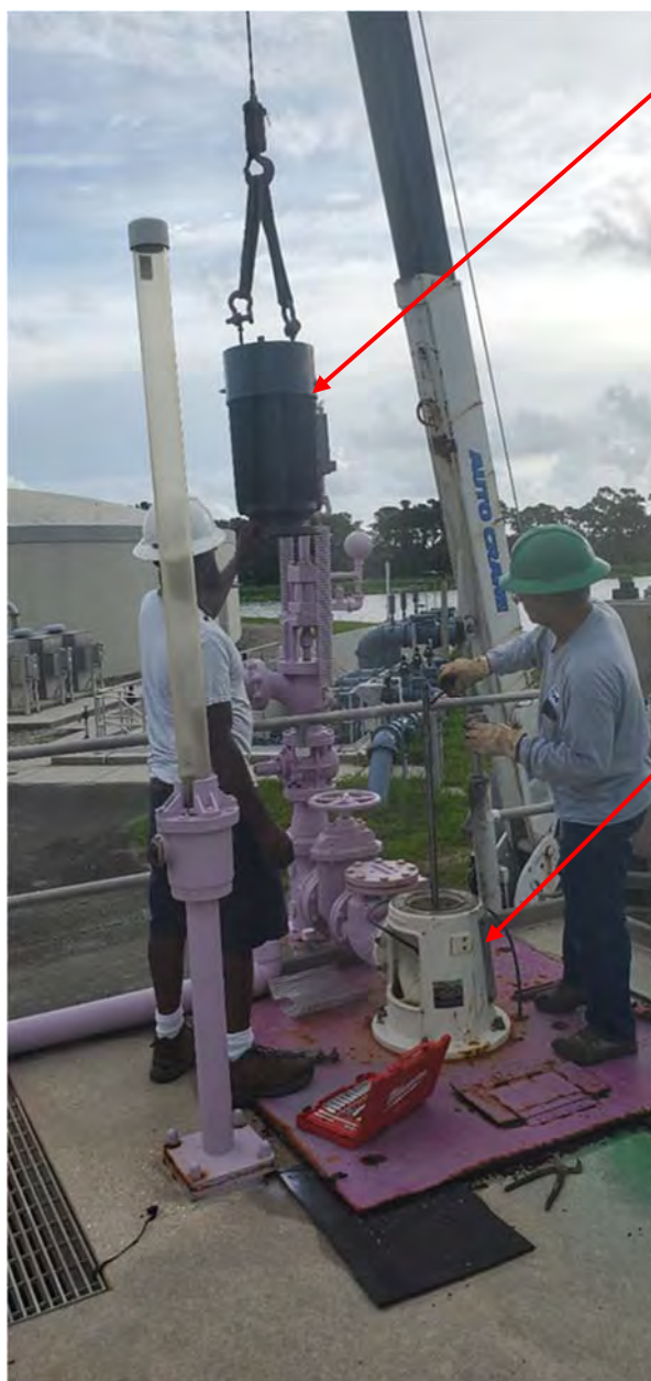
Maintenance Staff Replacing the A-Structure Service Water Pump Motor
