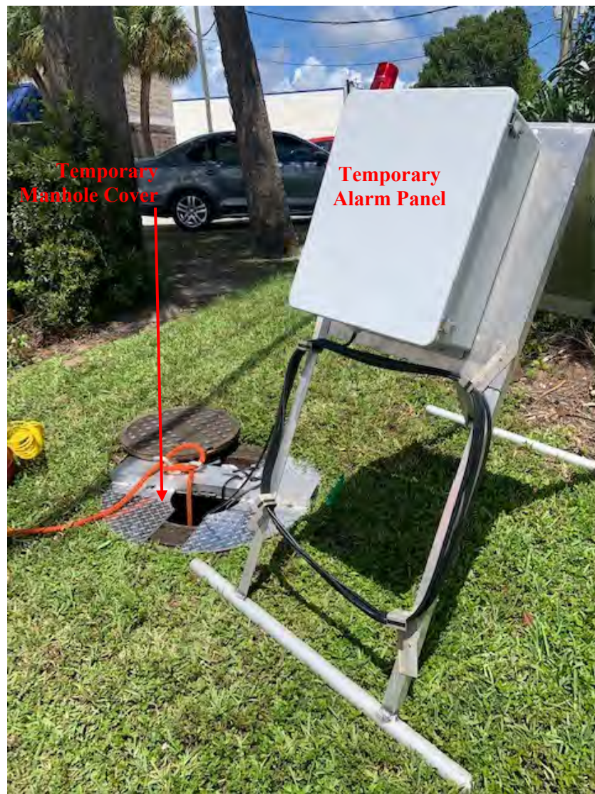
Lift Station No. 006 – Temporary Alarm Panel and Manhole Cover
