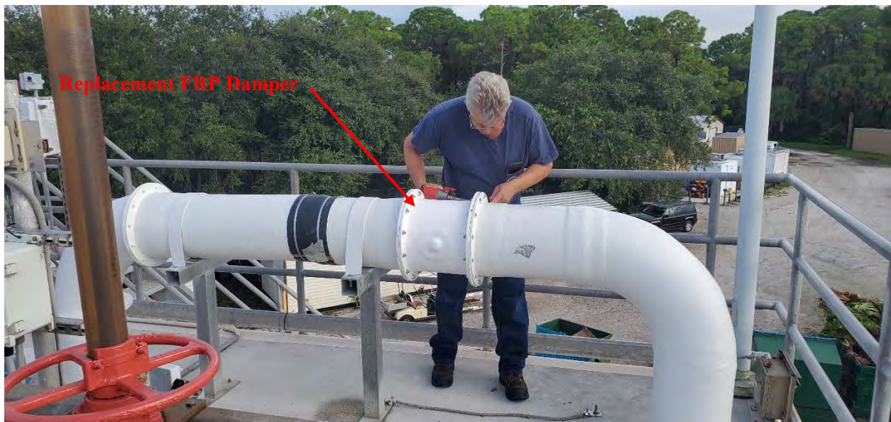
FRP Ductwork and Damper
