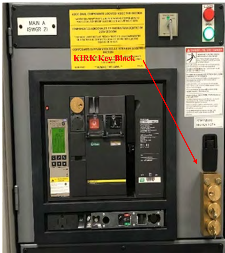
WWTF Electrical System – KIRK Key System Example
