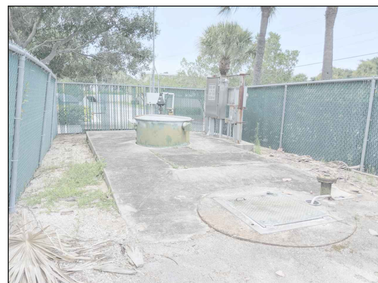
SITE PHOTO LOOKING NORTH
