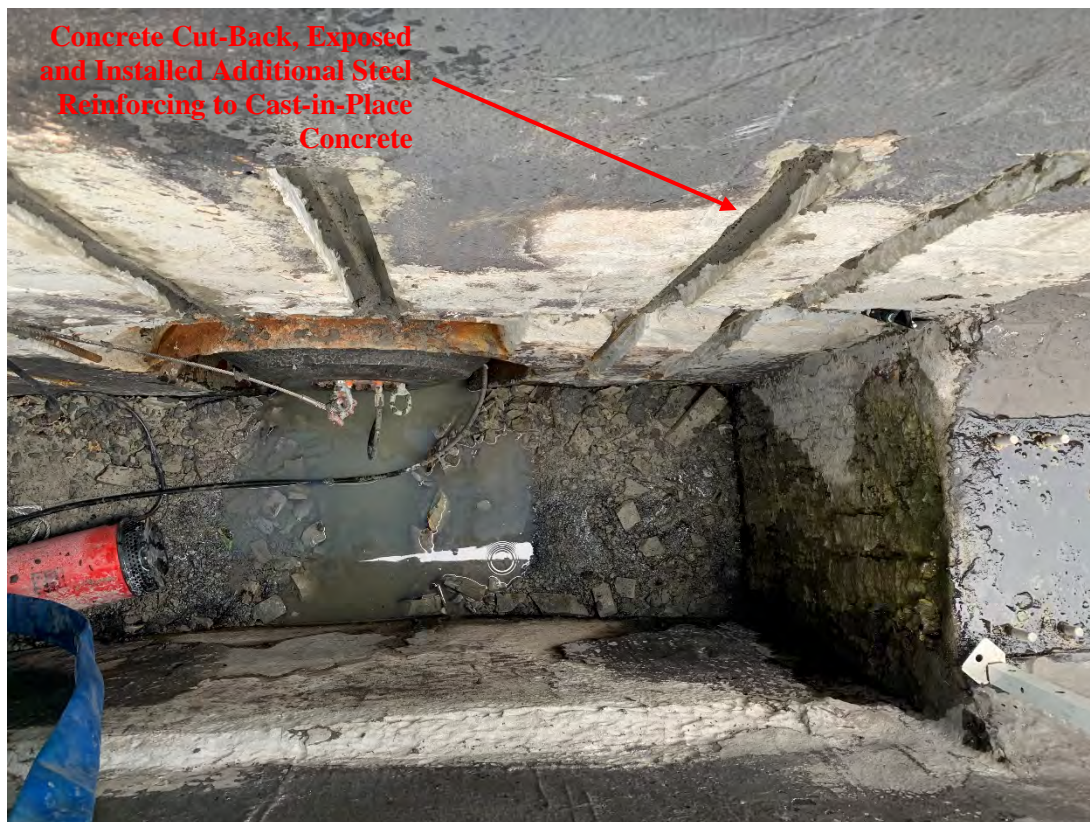
Clarifier No. 2 Effluent Box Repair – Photo No. 3
