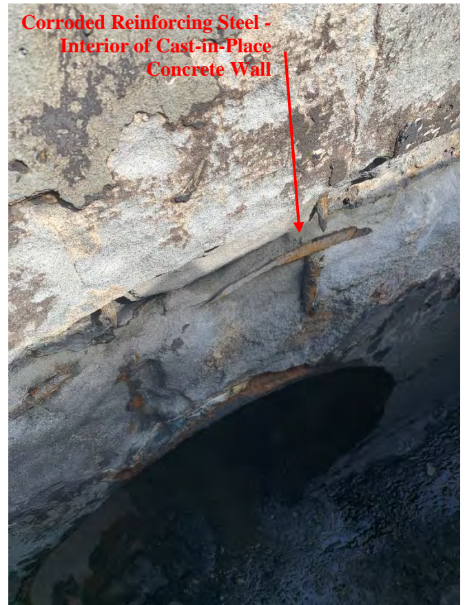
Clarifier No. 2 Effluent Box Repair – Photo No. 1
