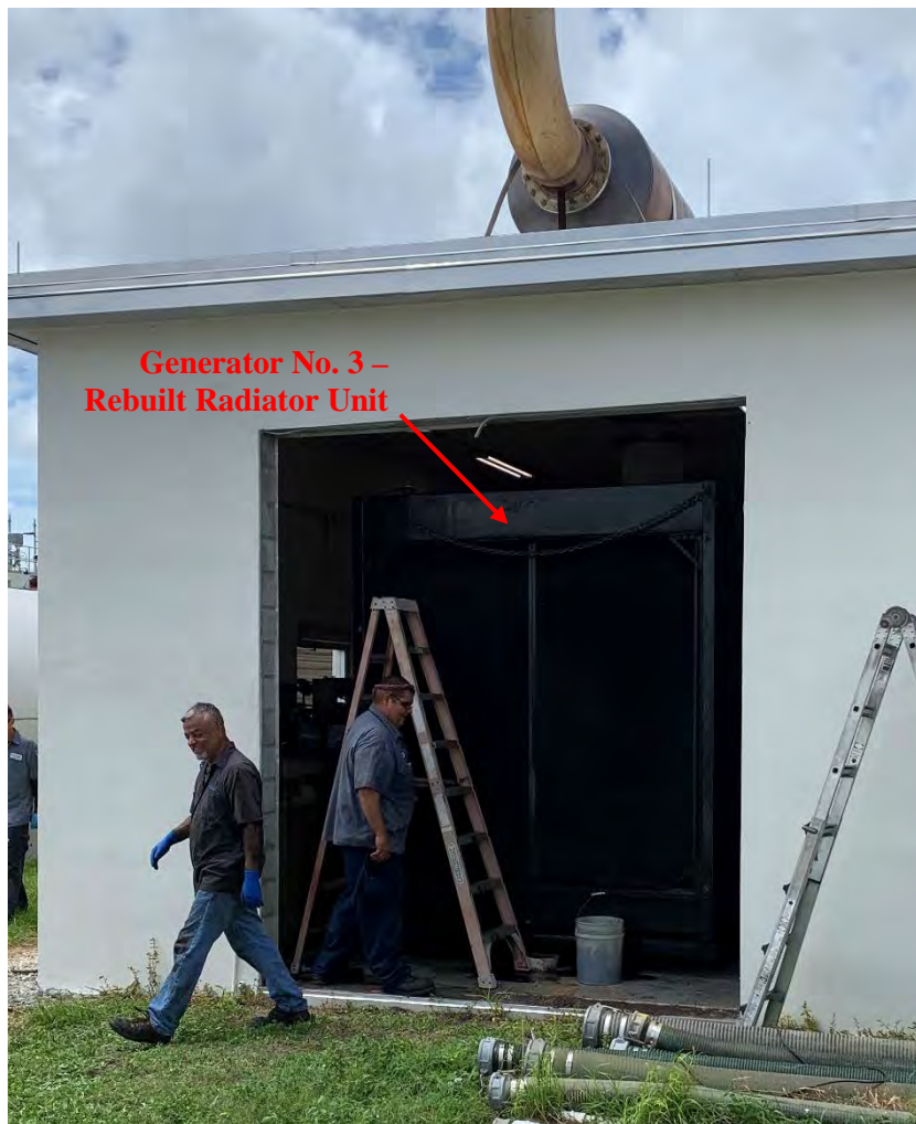
Generator No. 3 – Radiator Re-Core
