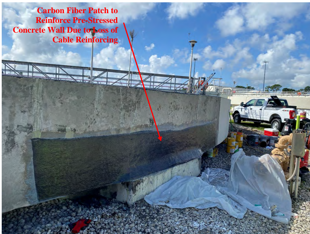
Clarifier No. 2 Effluent Box Repair – Photo No. 4
