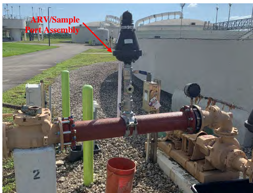
WAS Pump No. 2 - Piping Upgrades
