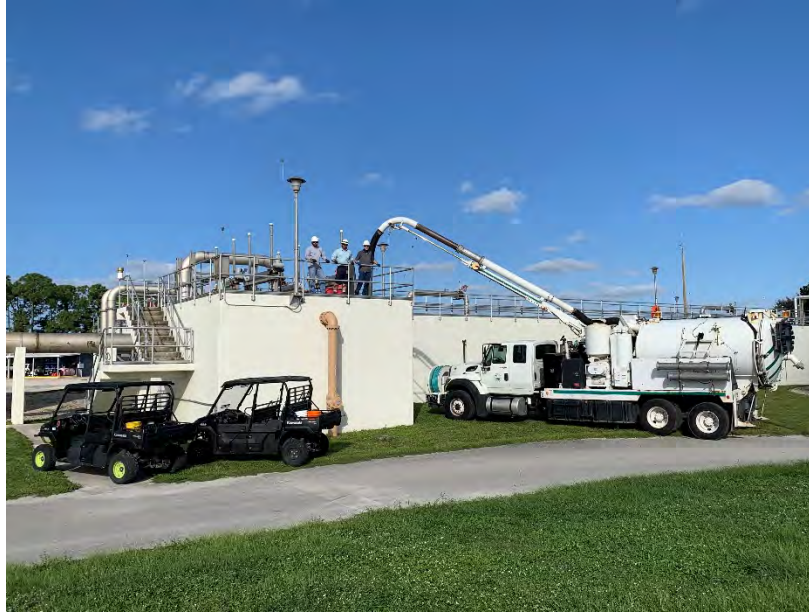
Clarifier No. 2 Flow Splitter Box Clean-Out
