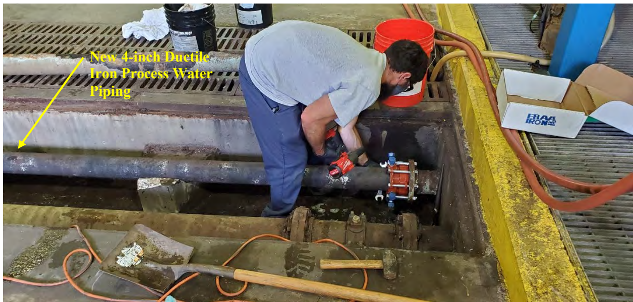
Replacement of Process Water Piping at Sludge Dewatering Facility – Photo No. 1
