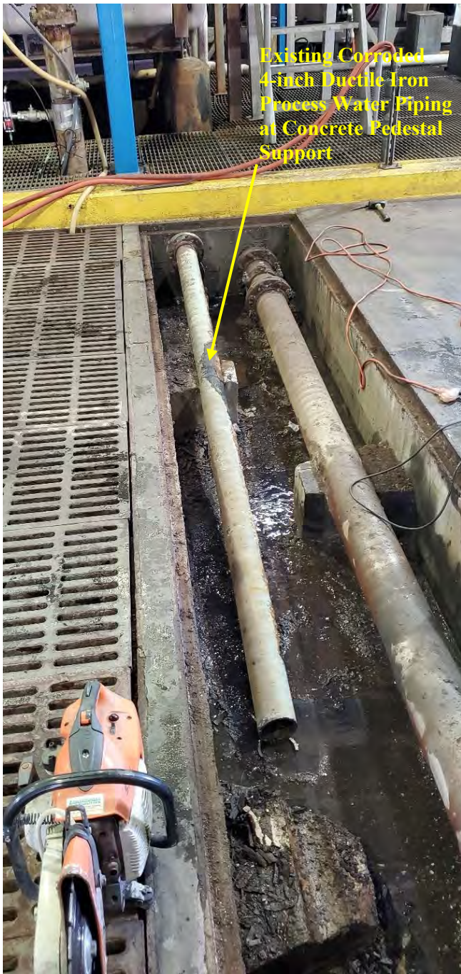
Replacement of Process Water Piping at Sludge Dewatering Facility – Photo No's. 2 and 3
