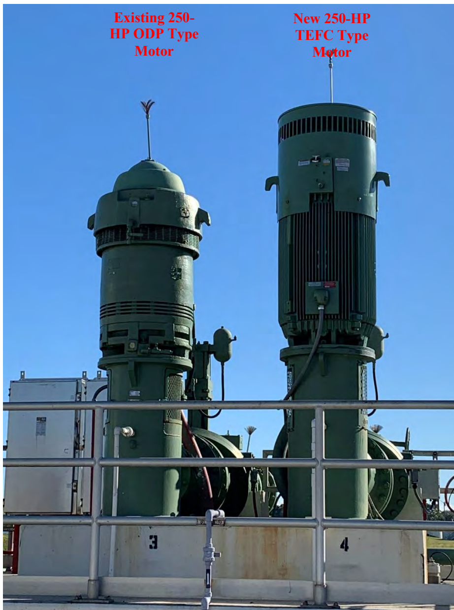
Replacement Vertical TEFC Motor at Injection Well Pump No. 4
