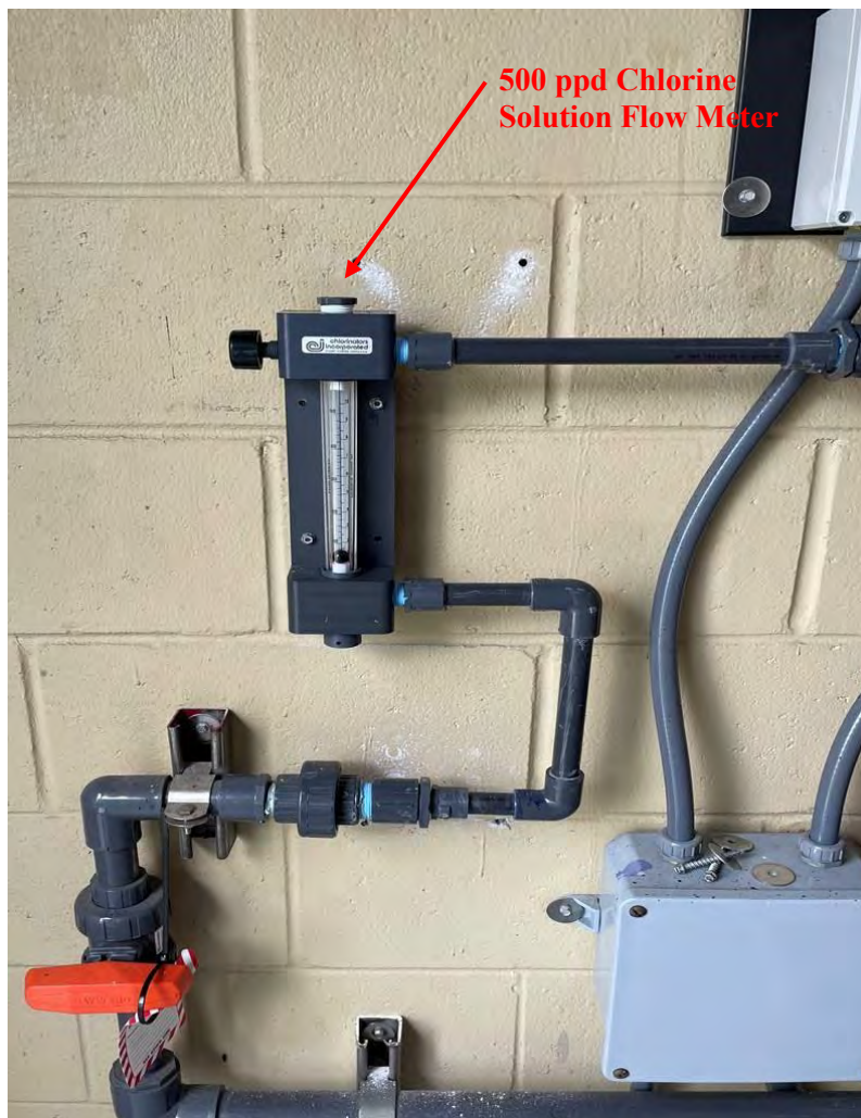
Clarifier Solution Flow Meter to Clarifier Units
