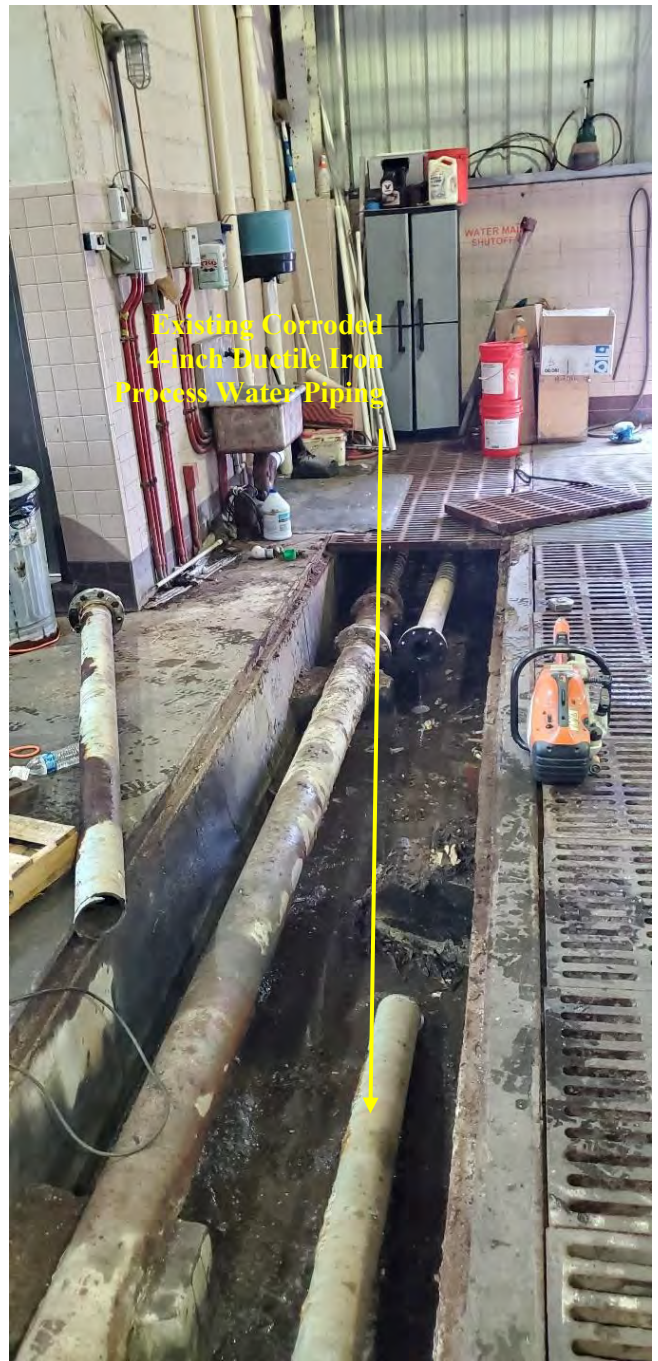
Replacement of Process Water Piping at Sludge Dewatering Facility – Photo No's. 2 and 3
