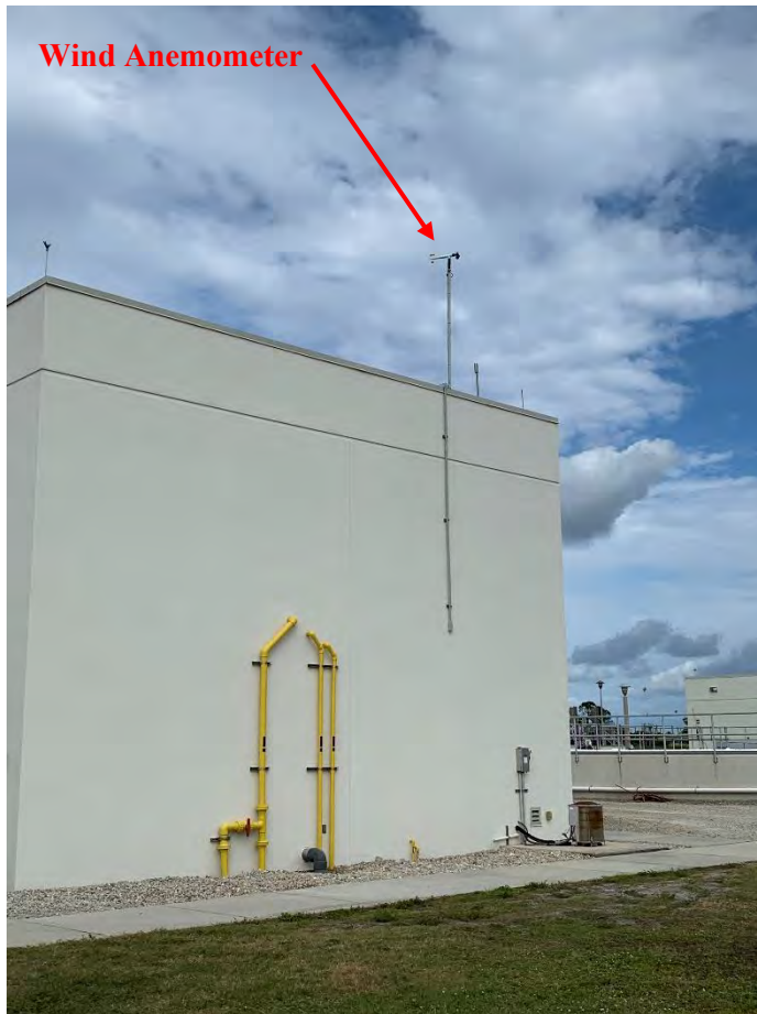
Chlorine Storage Building Wind Anemometer
