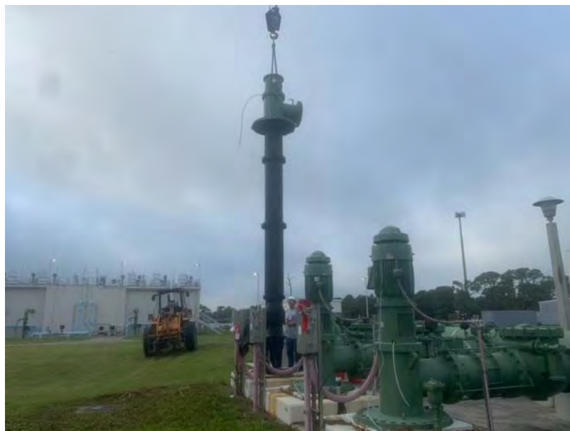
Removal of FPS No. 2 – Pump No. 1
