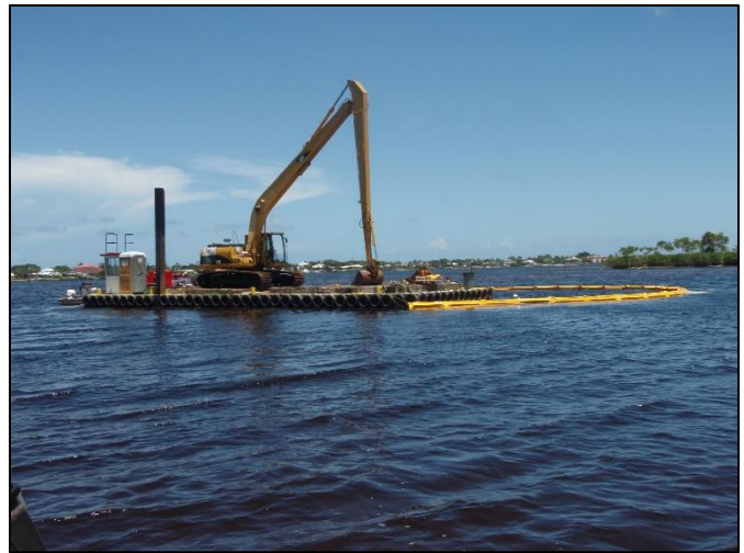
Photo 1. Image shows barge equipped with a long-arm excavator used to deploy shell material onto the oyster restoration sites during summer of 2010.
