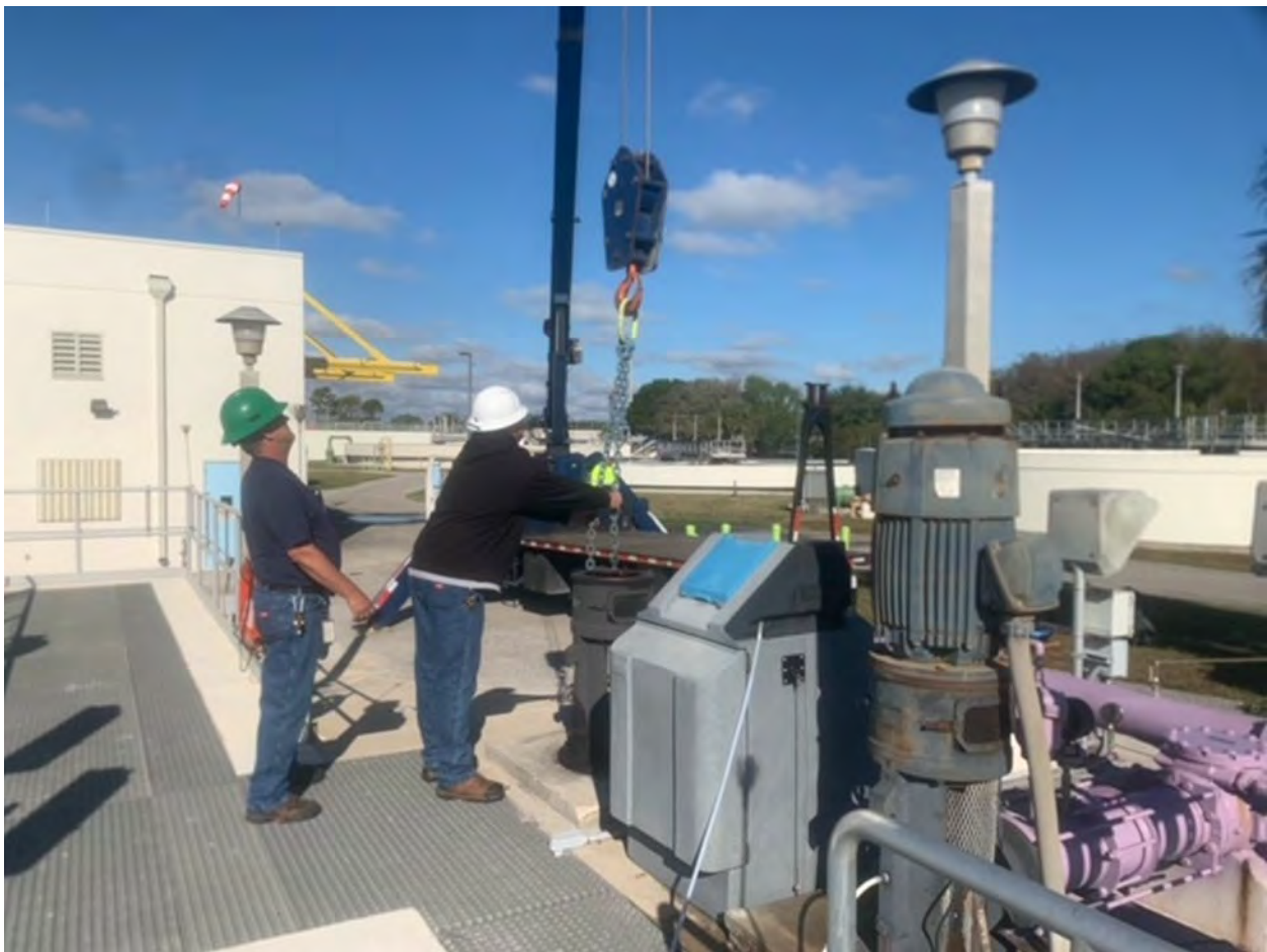
Replacement of Process Water Pump No. 1
