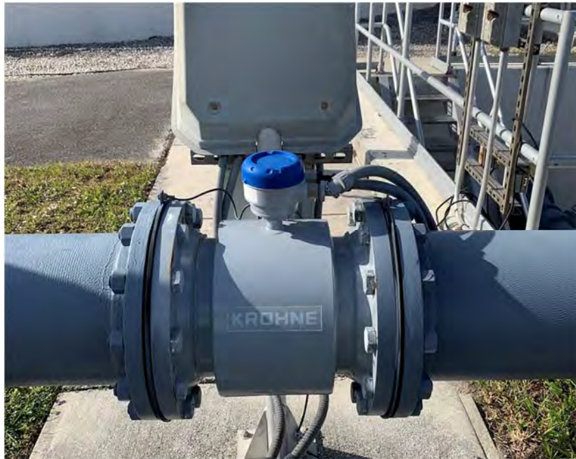
Inline Magnetic Flow Meter – Equalization Return
