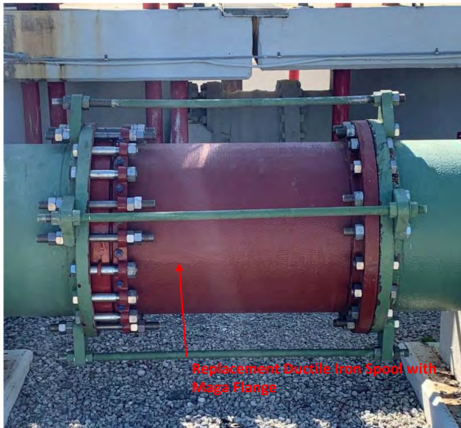
Replacement Coupling with Mega-Flange to Address Drip Leak
