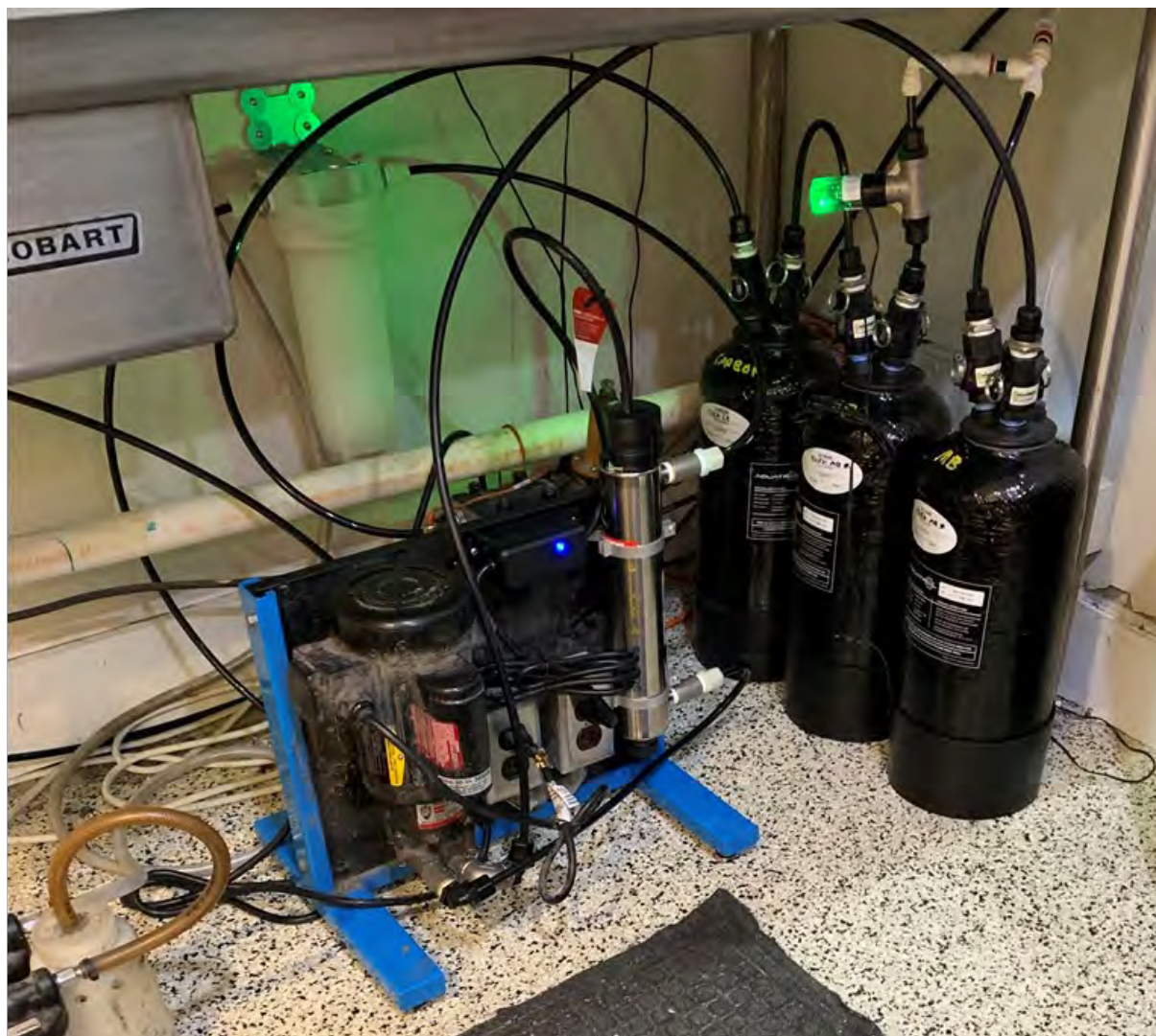
Operations Laboratory – Replacement DI Water System
