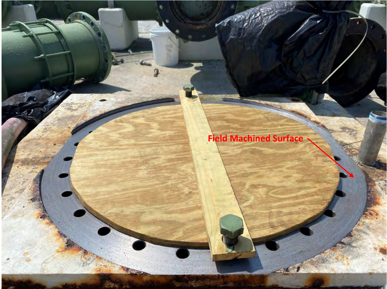
Final Field Machined Level Pump Base Plate
