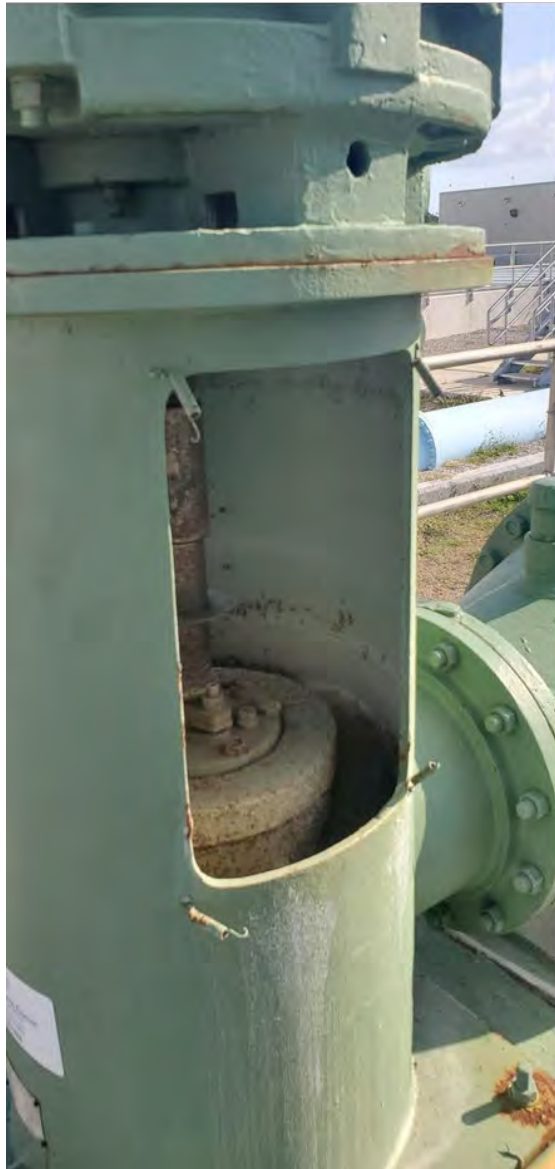
Injection Well Pump Drive Coupling – Safety Guard Replacement
