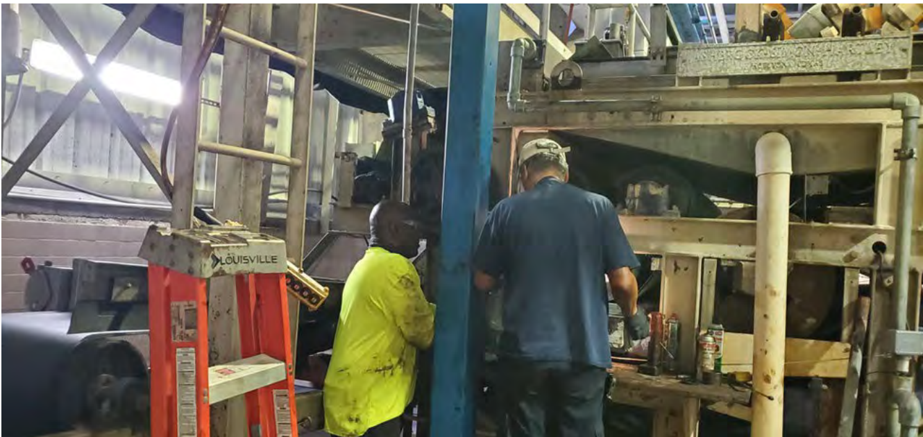
Maintenance Team Making Repairs to Belt Filter Press Unit Drive
