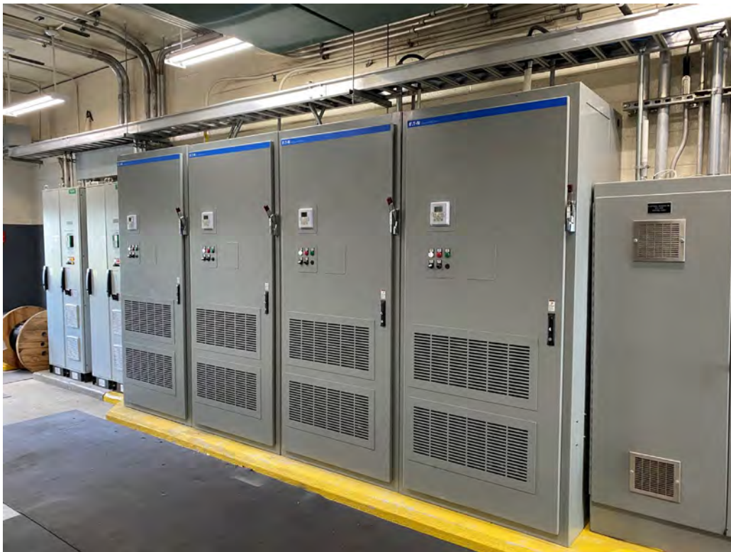
Replacement DIW Variable Frequency Drives
