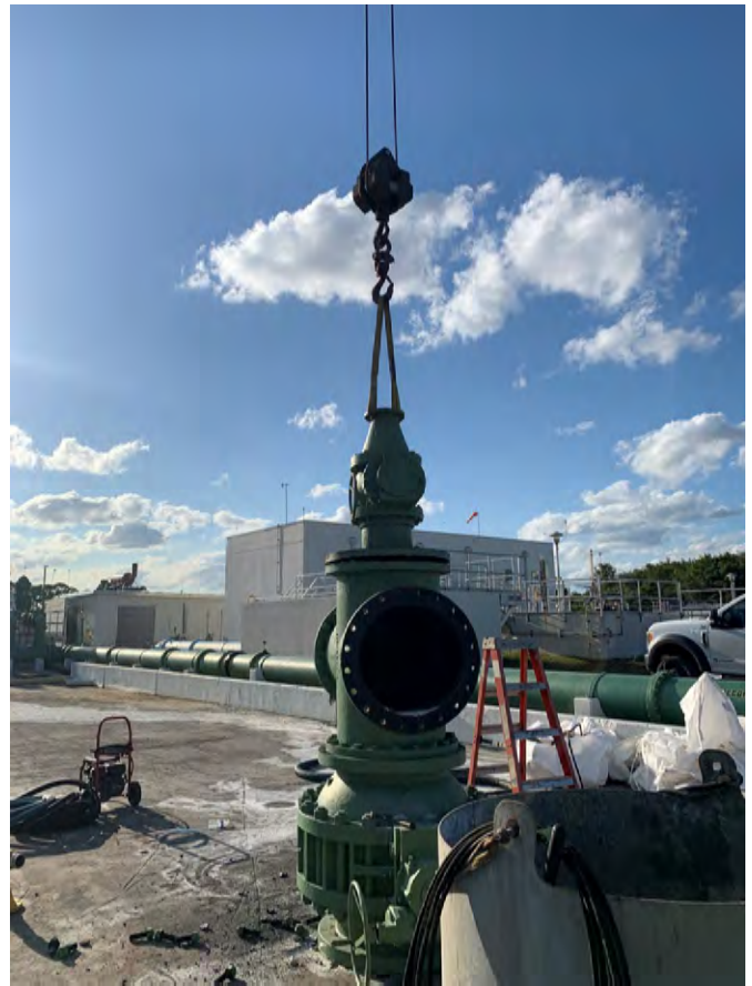
Removal of DIW Wellhead Piping
