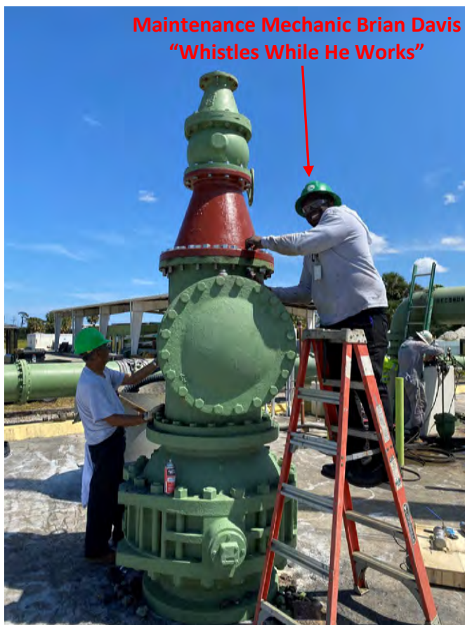
Replacement Reducer on DIW Wellhead
