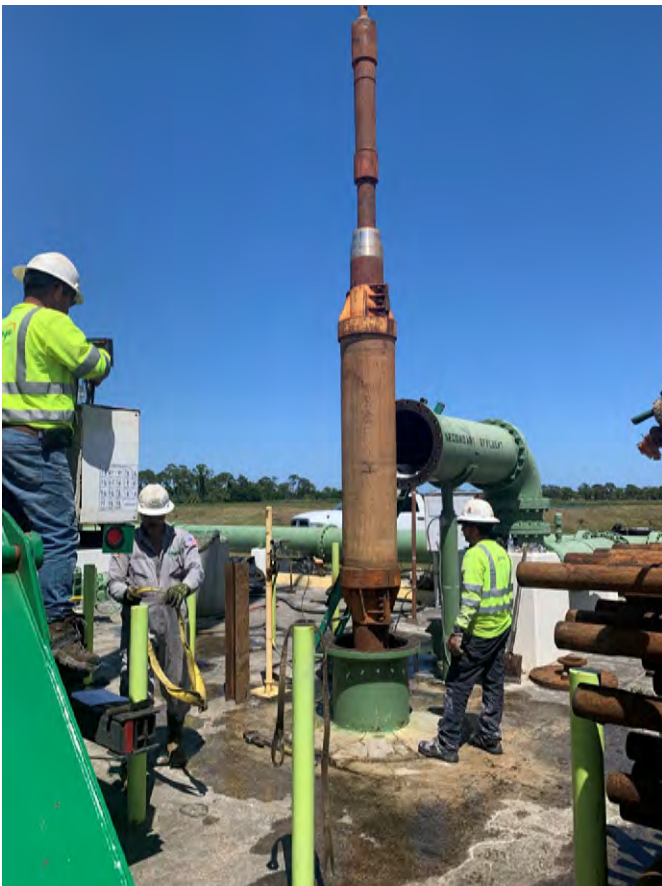
Install of Inflatable Packer for Casing Pressure Test
