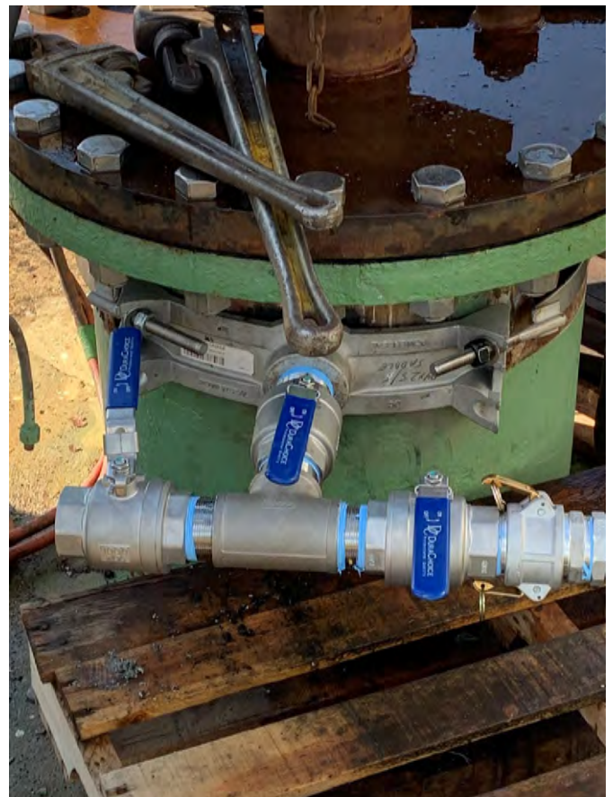
Replacement Pressure Transmitter Saddle
