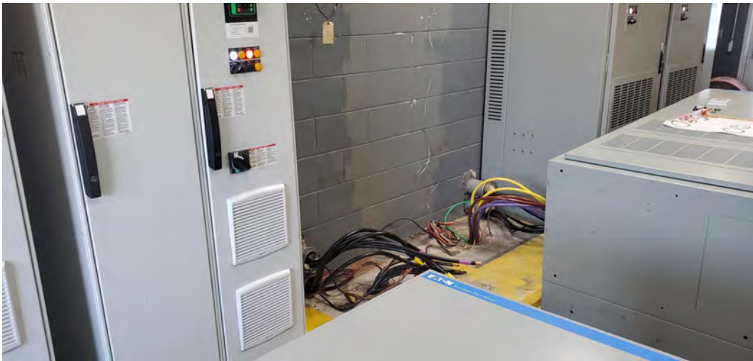
Removal and Installation of DIW Variable Frequency Drives
