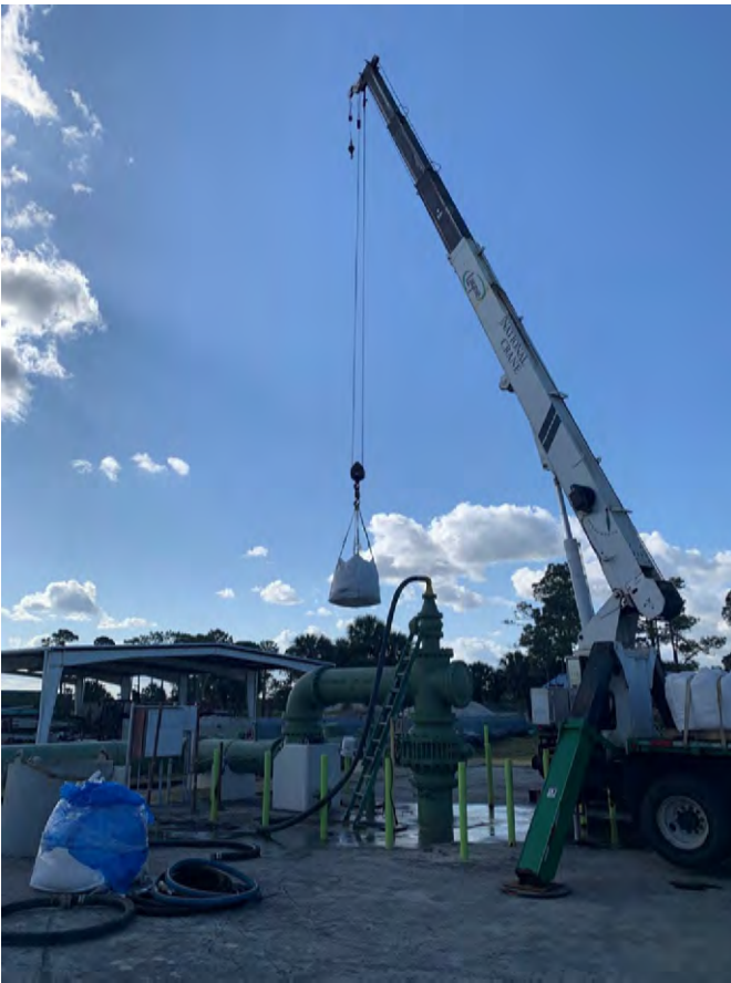
Injection of Brine Solution for Salt Plug
