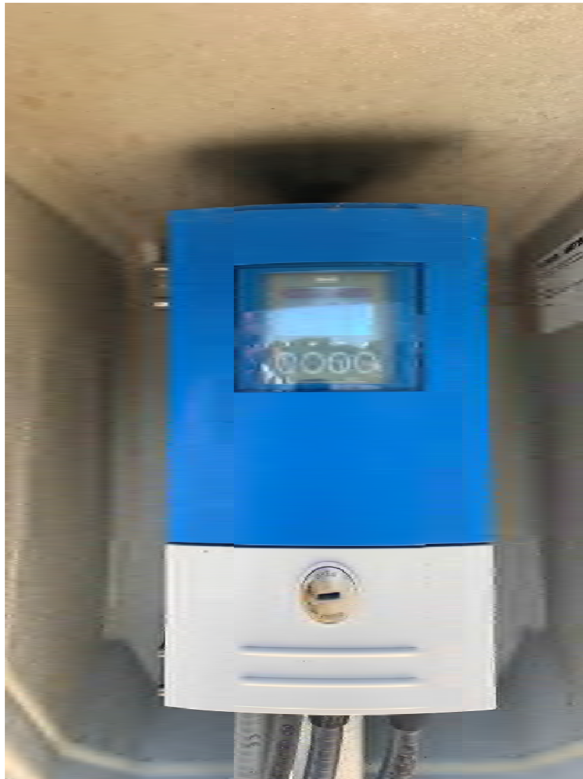
Inline Magnetic Flow Meter Transmitter – Deep Bed
