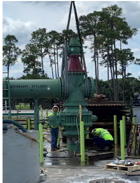
Reinstallation of Deep Injection Wellhead Piping
