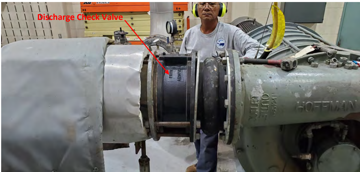
Process Air Blower – Discharge Check Valve Replacement
