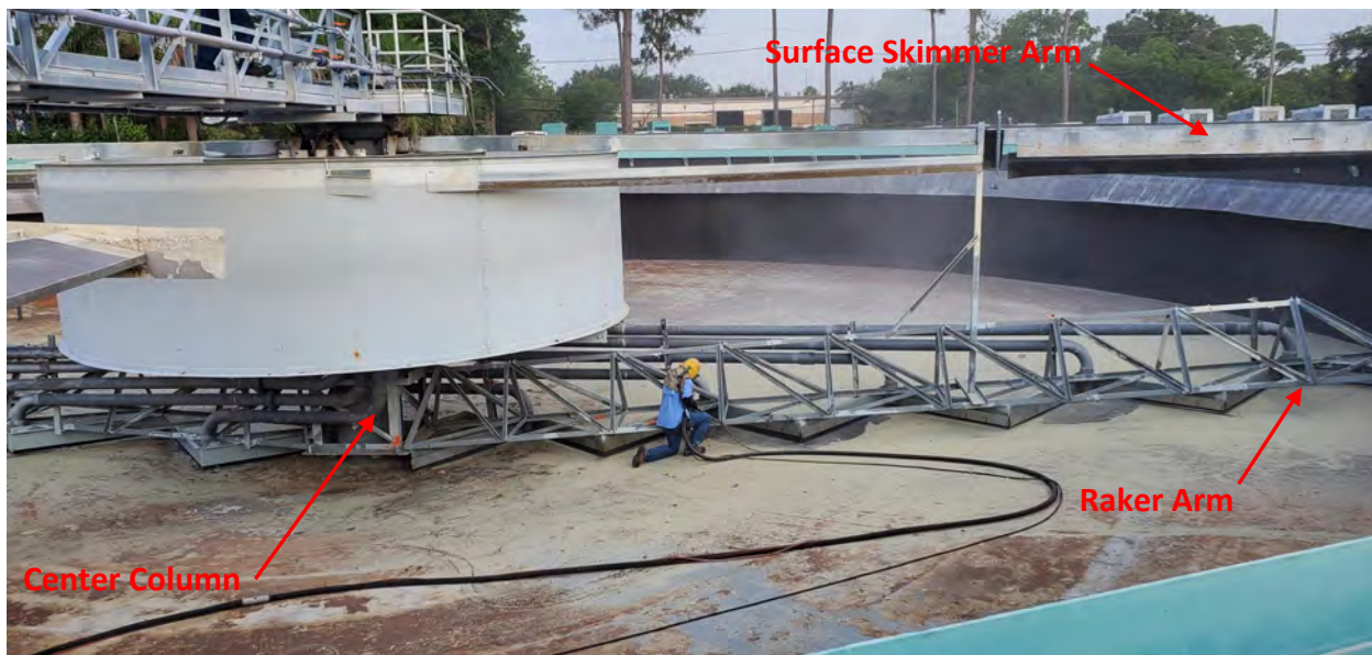
Clarifier No. 1 – Surface Preparation and Coating Repairs
