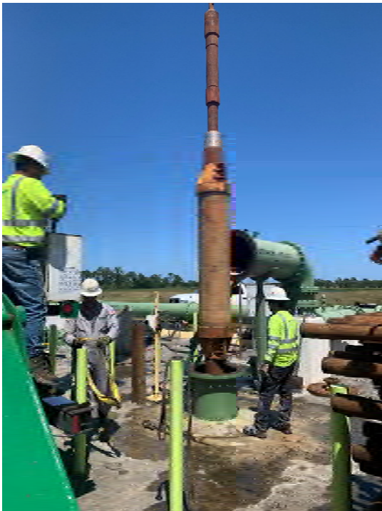
Installation of Packer for DIW Pressure Test
