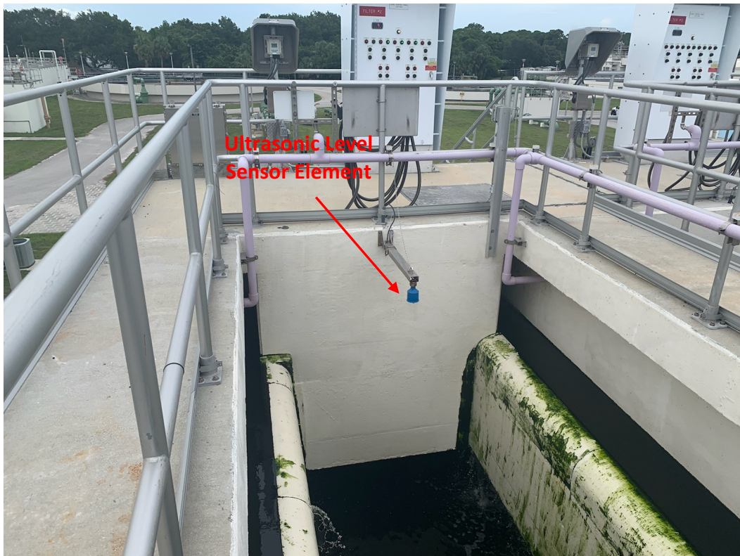
Deep Bed Filter Unit – Ultrasonic Level Sensor
