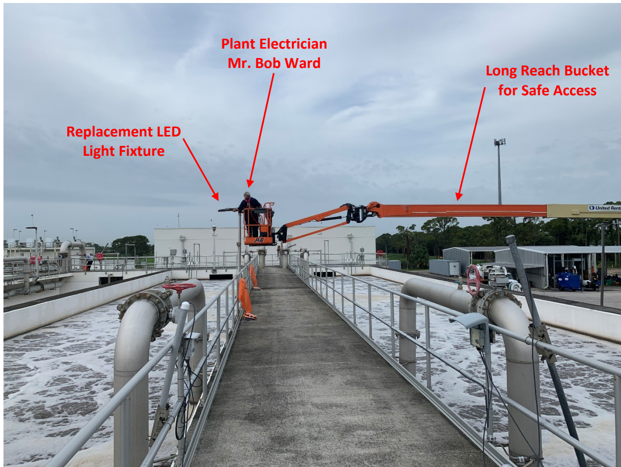
Installation of LED Light Fixtures at Aeration Basin
