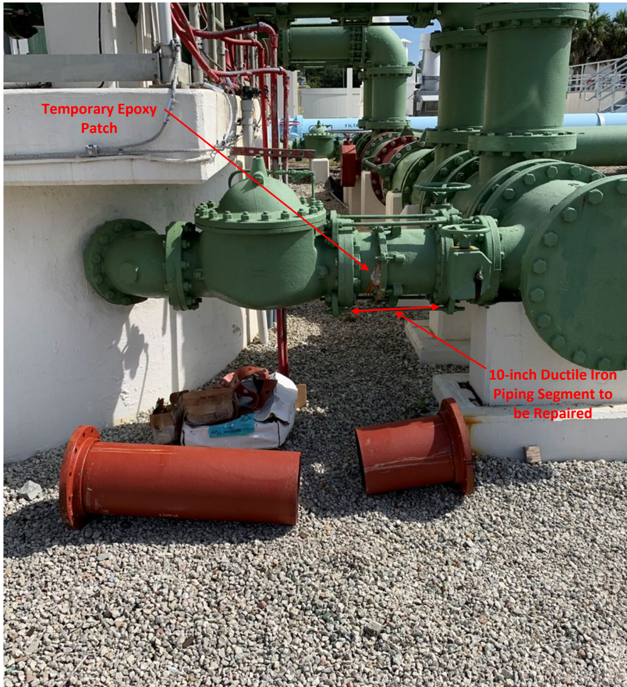
Injection Well Pump Station Piping Repair – Photo 1
