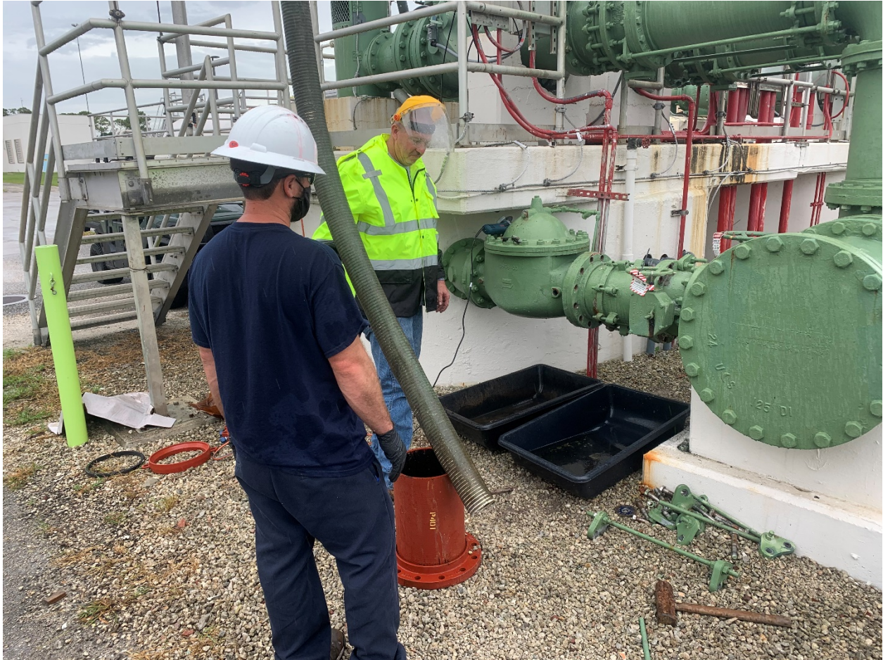
Injection Well Pump Station Discharge Piping Repairs
