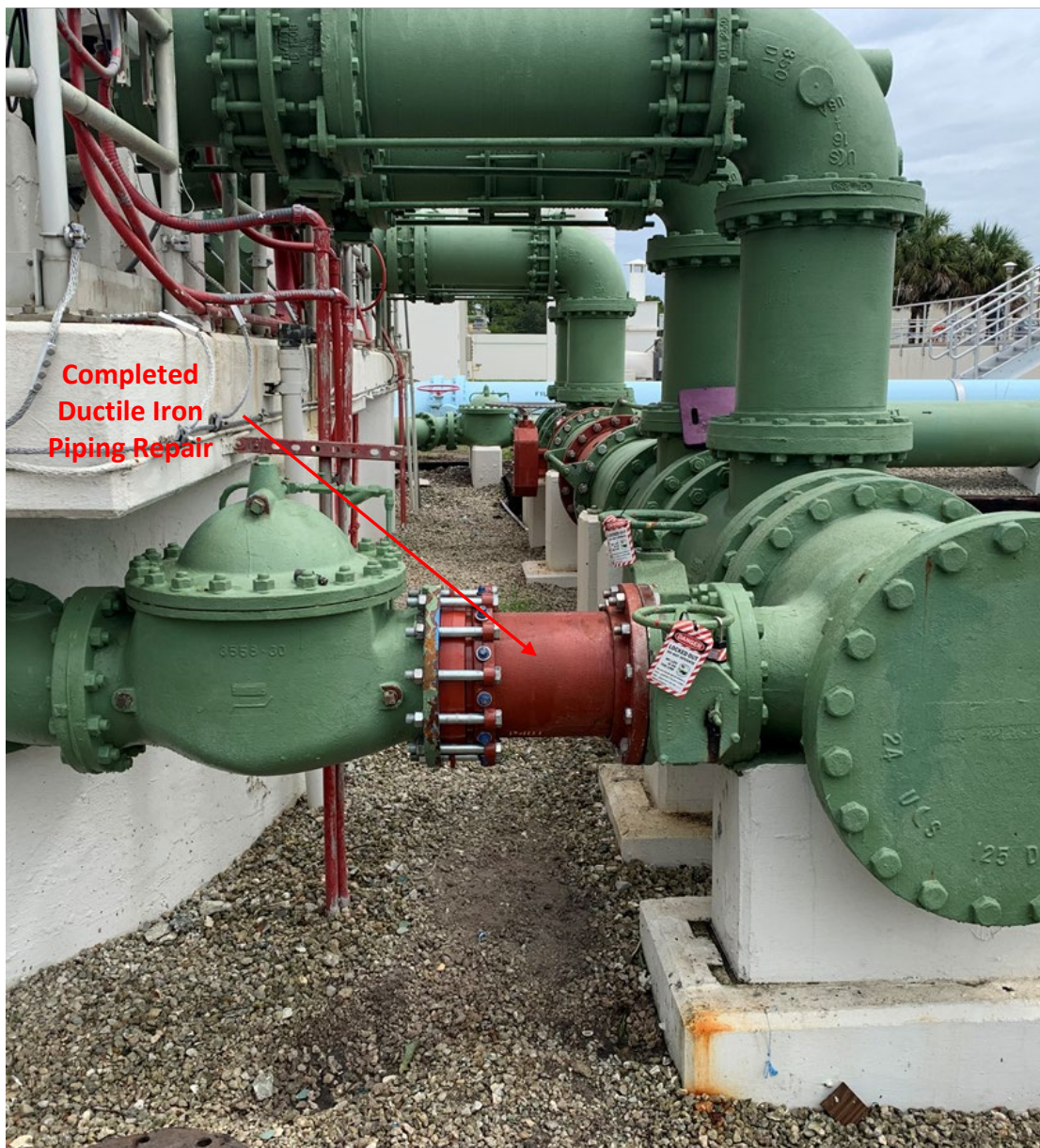
Injection Well Pump Station Piping Repair – Photo 2
