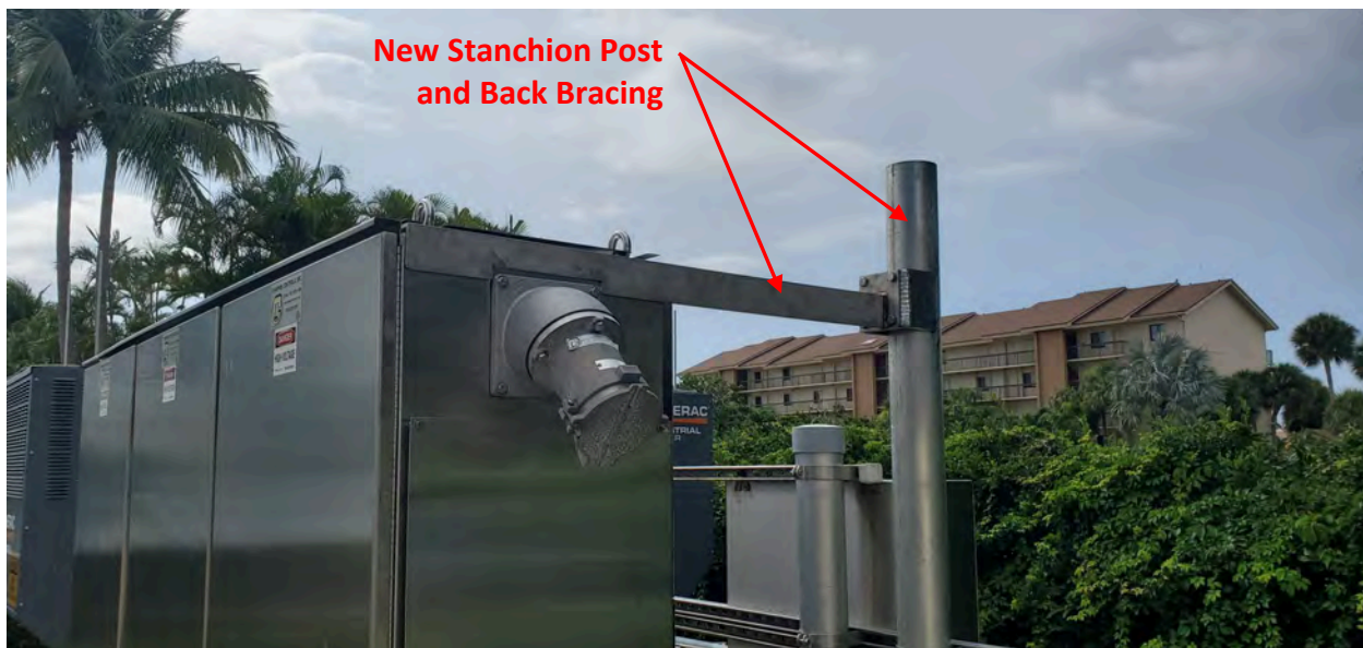
Lift Station No. 114 – Electrical Panel Improvements – Photo No. 2
