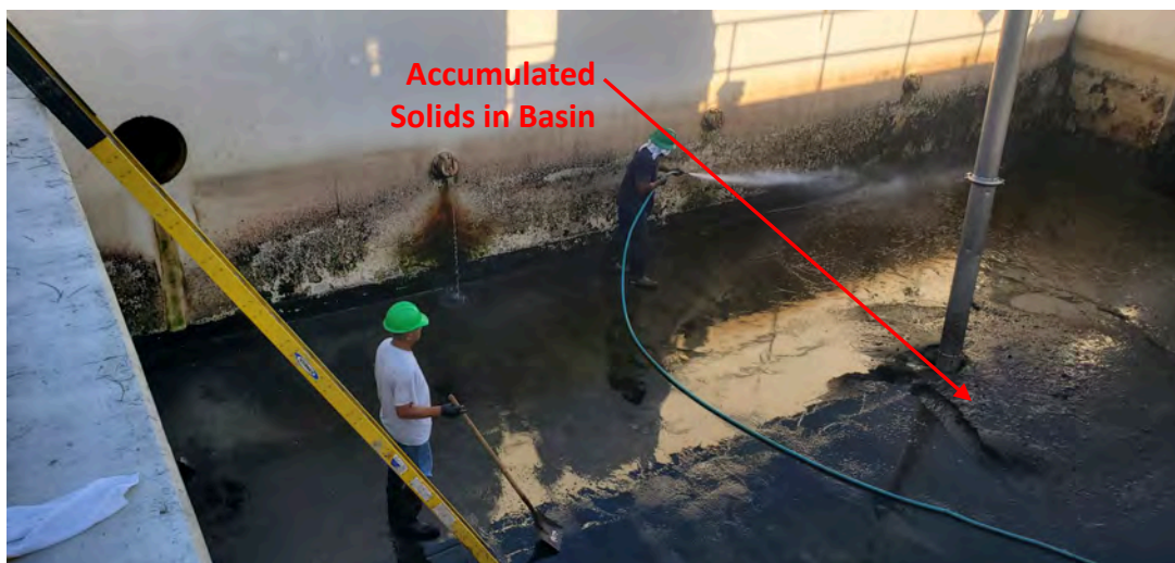
Filter Backwash Basin Cleaning – Photo No. 2
