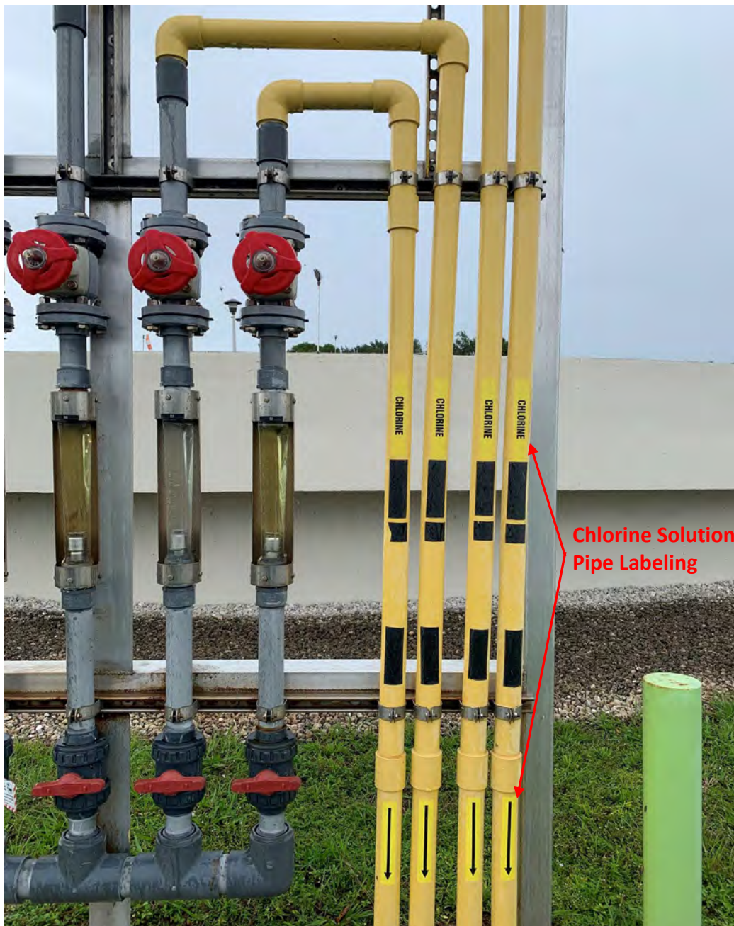
Clarifier Chlorine Solution Tree - Feed Piping Labeling
