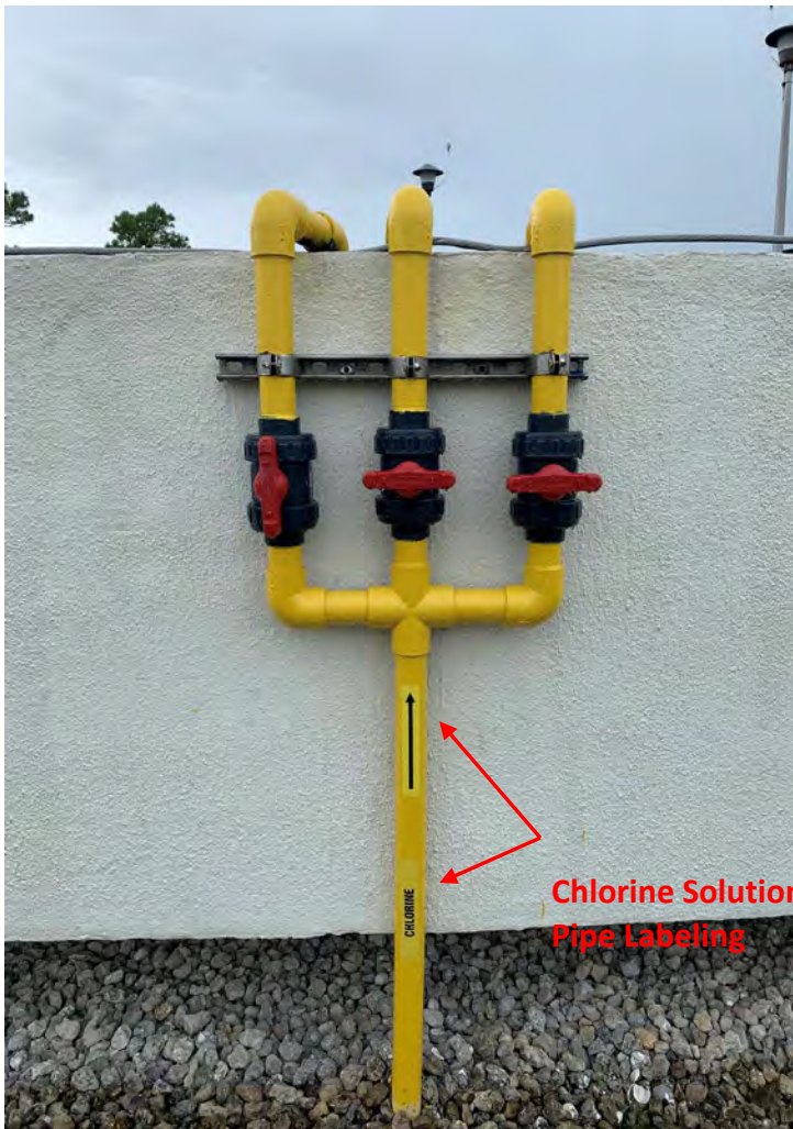
Clarifier Chlorine Solution - Feed Piping Labeling
