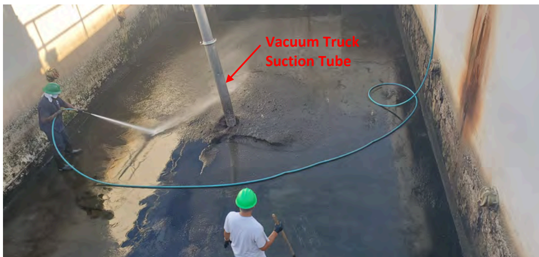
Filter Backwash Basin Cleaning – Photo No. 1
