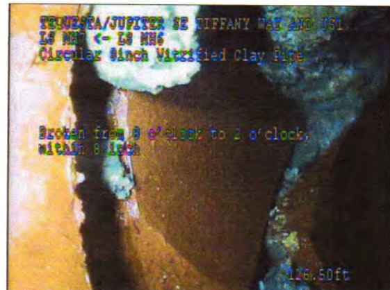
65811e3f-fc6d-4d26-9801-179dc9d5e888_20200213_124517_541.jpg, 00:03:38, 126.50ft Broken from 8 o'clock to 2 o'clock, within 8 inch
