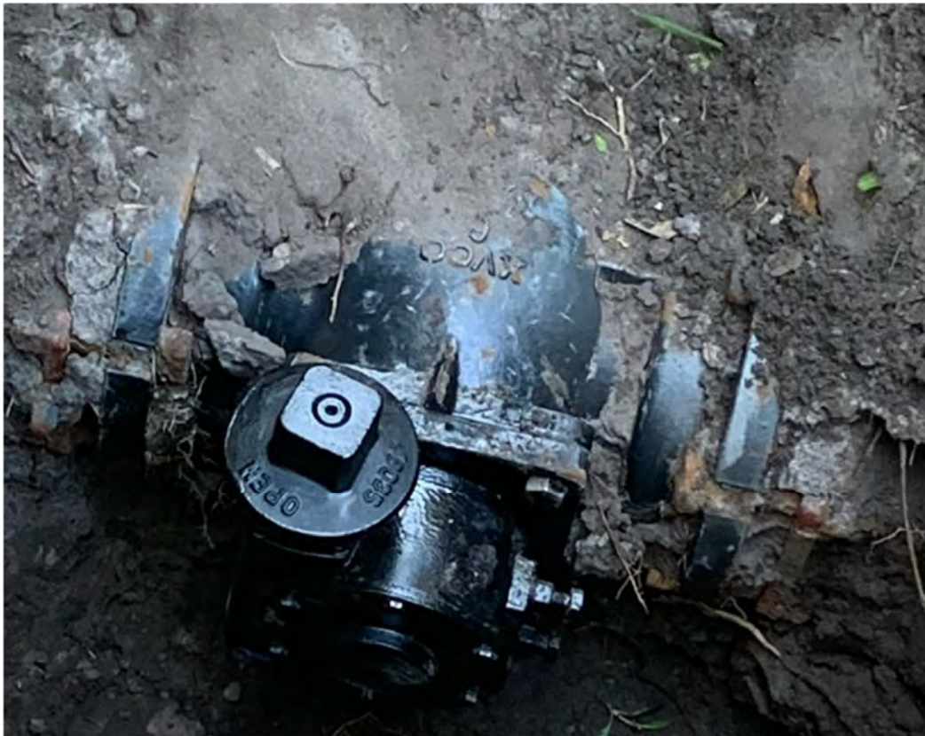
Replacement Actuator on Buried Plug Valve
