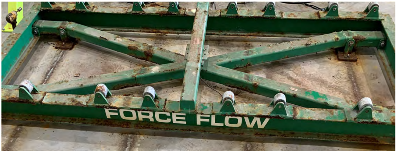
Existing One-Ton Chlorine Cylinder Scale
