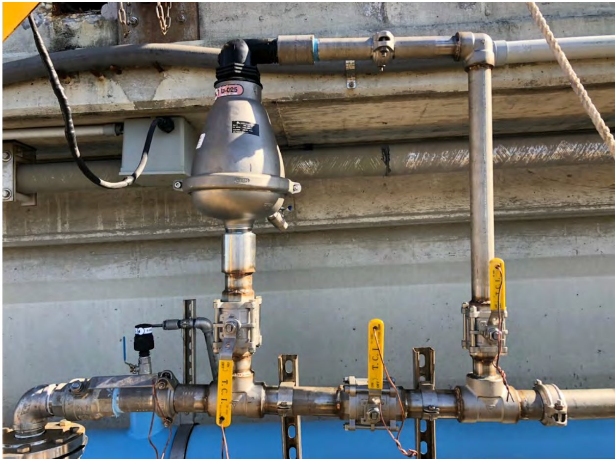
Alternate A1A Aerial Force Main - Shop Fabricated ARV and Bypass Piping Assembly
