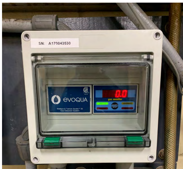
Chlorine Leak Detector Analyzer
