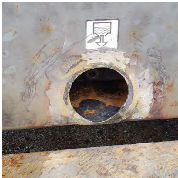
Existing Opening for Base Containment Plug
