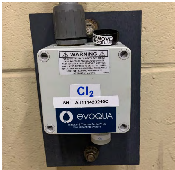
Chlorine Leak Sensor Unit
