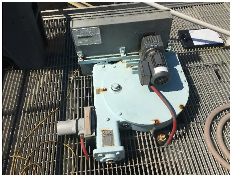
Photo 6: Clarifier Drive, Corrosion is Apparent beneath the Grating
