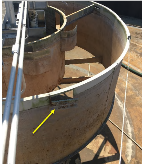
Photo 7: Degraded Scum Window Flaps
