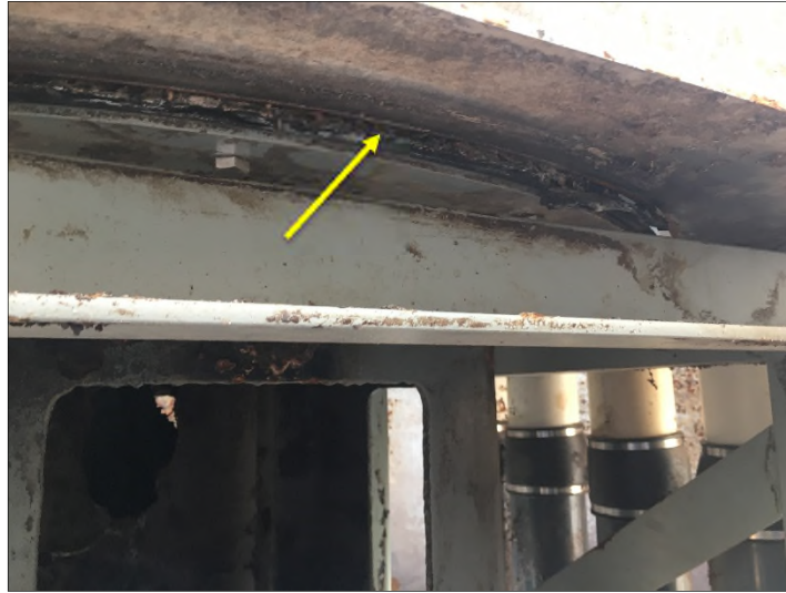
Photo 3: Deteriorated RAS Box Seal
