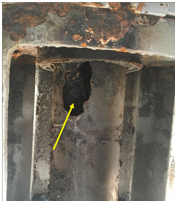
Photo 2: Corroded RAS Pipe
