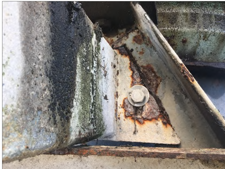
Photo 4: Corroded Skimmer Arm Connections, Typical of 4 Locations
