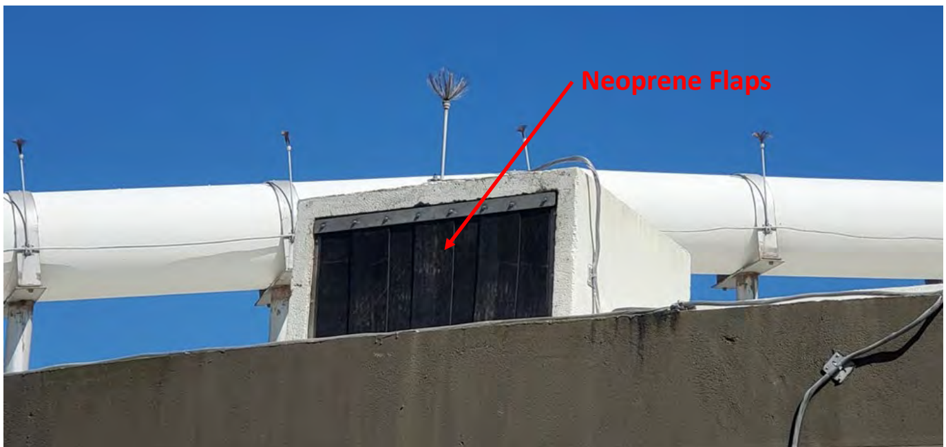
Sludge Storage Tank Vent Modifications – Picture No. 4
