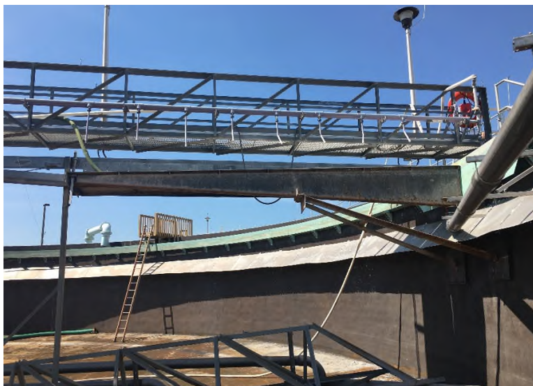
Photo 12: View of Existing Galvanized Steel \frac{1}{2} Radius Scum Trough
