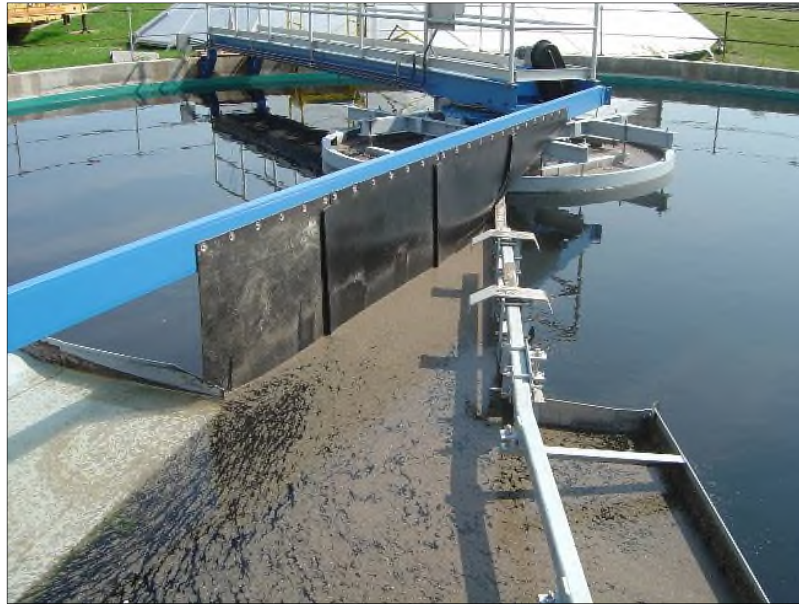
Photo 13: View of a Typical Anti-Rotational Scum Baffle at another Plant
