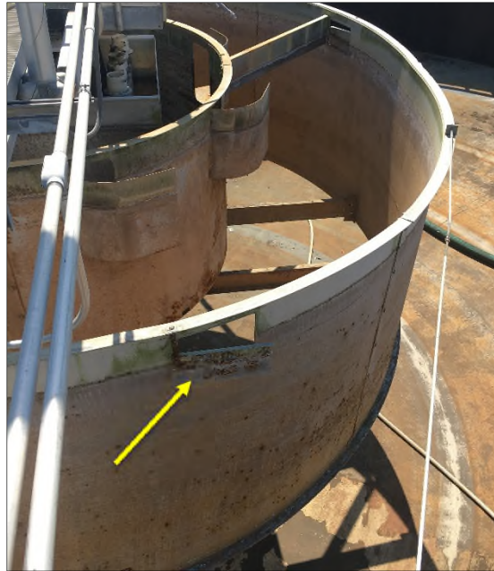
Photo 7: Degraded Scum Window Flaps
