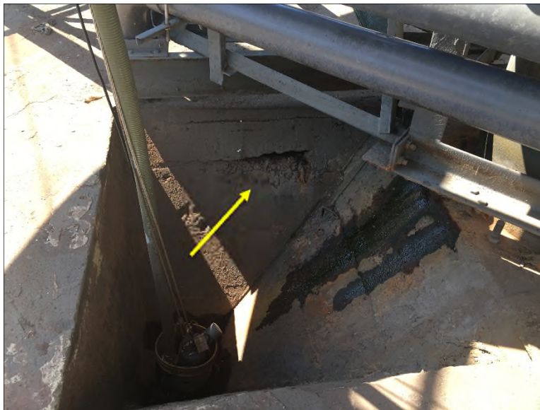
Photo 10: View of Gap at Construction Joint between Sludge Hopper and Tank Slab
