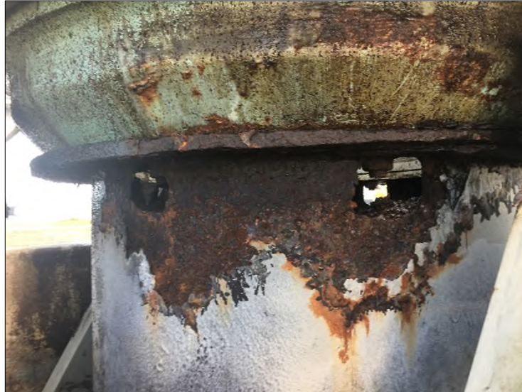
Photo 5: Corroded Connection of Center Column to Drive
