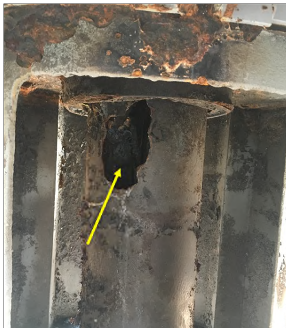
Photo 2: Corroded RAS Pipe
