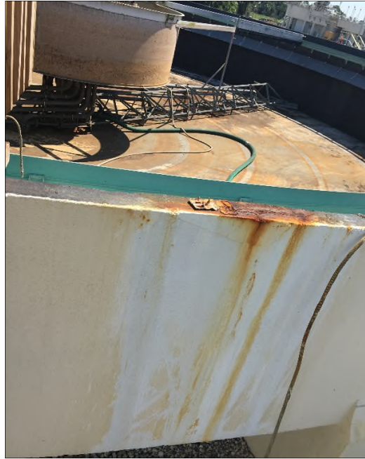
Photo 11: View of Spalled Concrete and Corrosion at Top of Prestressed Concrete Tank
