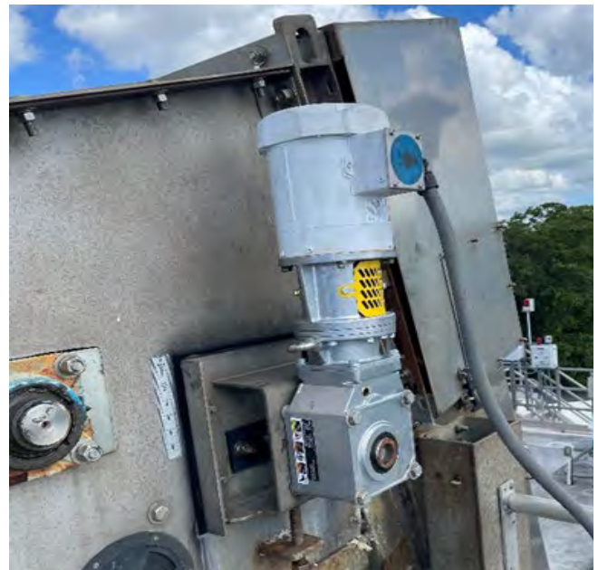
Final Gearbox and Drive Replacement Photos
