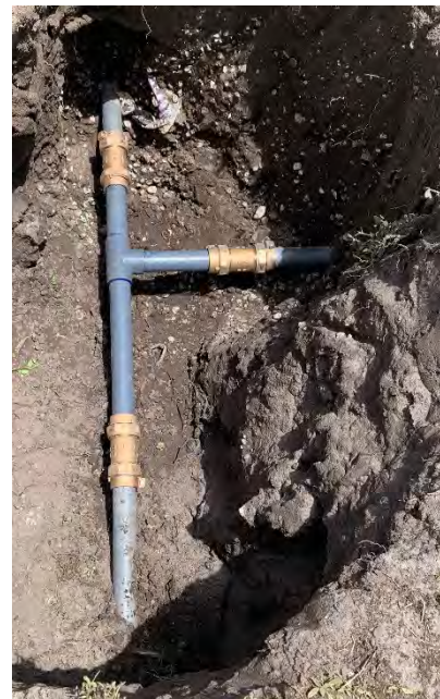
Process Water Piping Repair
