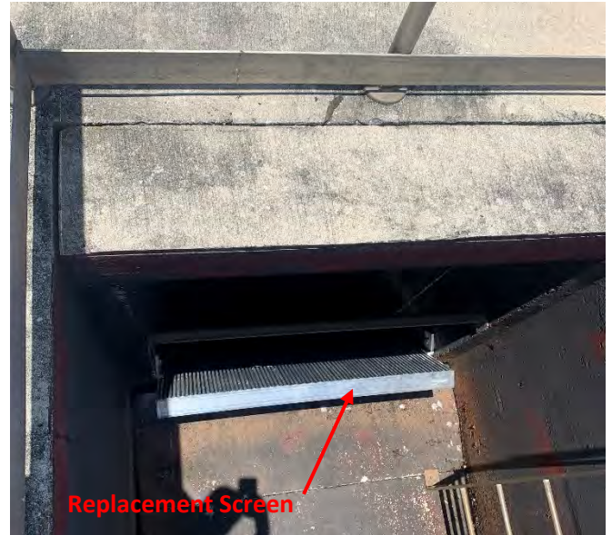
IW Replacement Screen - Installed
