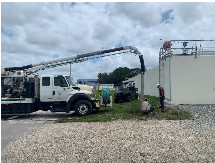
Process Water Piping Excavation
