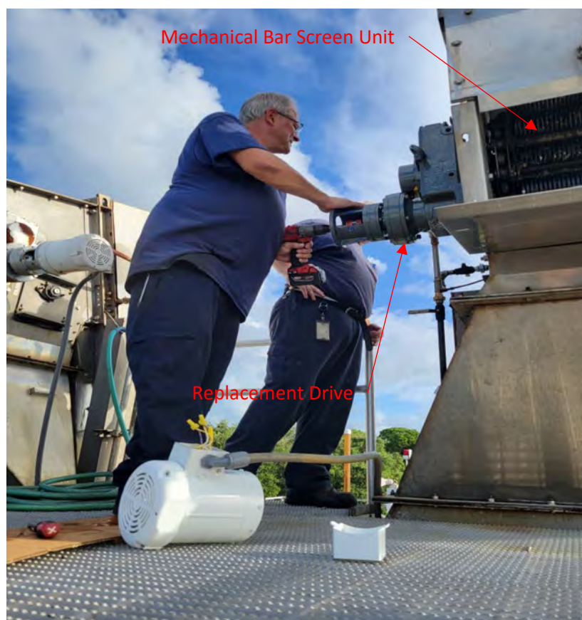
Replacement of Mechanical Bar Screen Drive Motor
