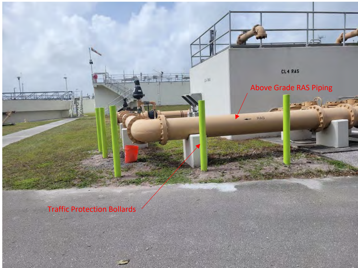
New Traffic Protection Bollards at RAS Pump Station
