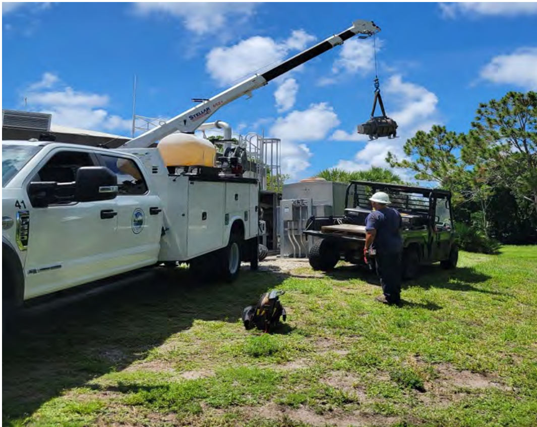
Sludge Storage Tank - Process Air Blower Replacement
