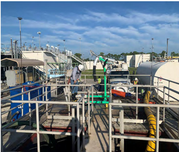
IW Screen Structure – Confined Space Entry
