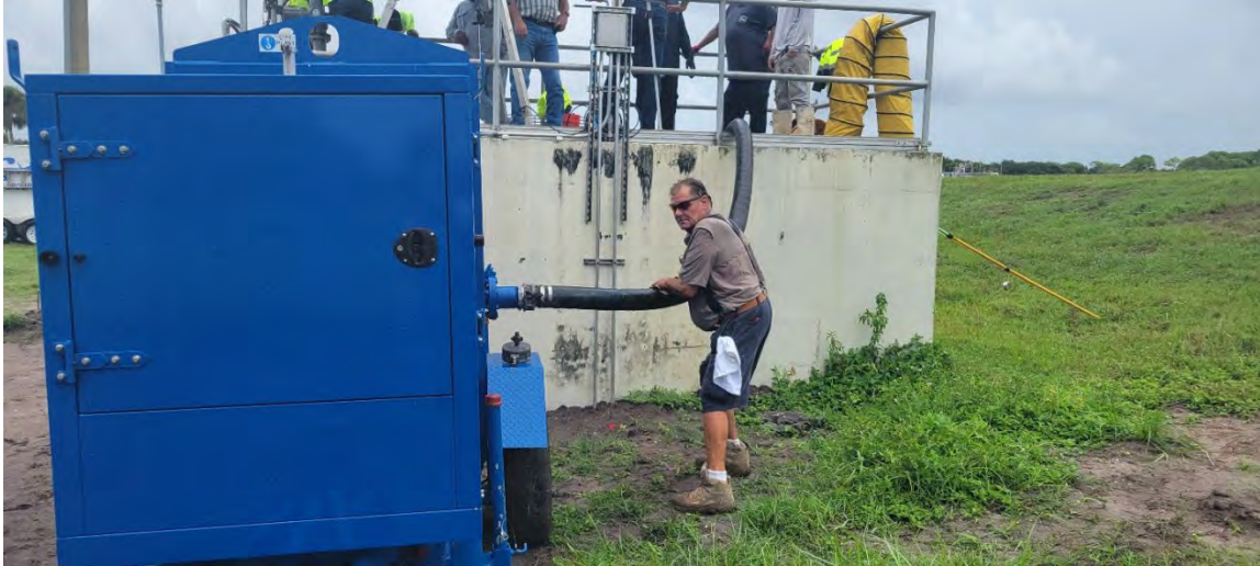
Temporary Diesel Pump Setup at B-Structure
