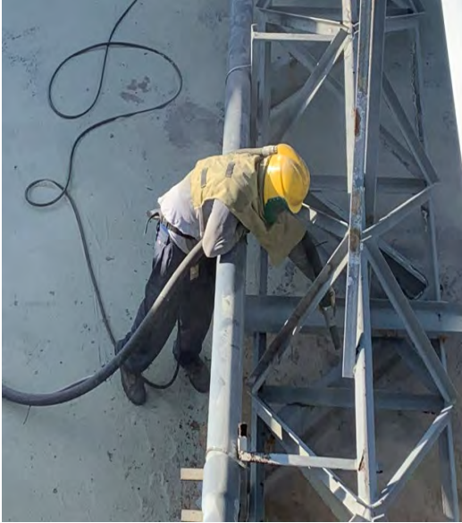
Pictured at left: Brian Davis is donning a breathing air hood while blasting the rake arm in clarifier 3. At right: Kemm Peebles documents activity on the confine space permit while observing Brian. The rake arm would be painted at a later date.
