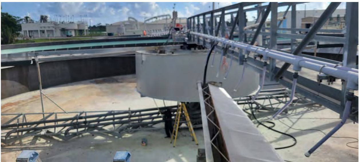
Clarifier No. 3 – Surface Preparation and Re-Painting of the Mechanism
