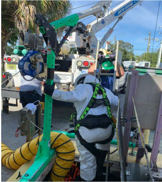
Pictured at left: Jonathan Martins is entering L/S 02 as Ben McTigue supports the confined space entry. At right: Dwayne Martin documents activity on the confined space permit while Ben keeps an eye on Jonathan as he inspects the critical areas of the L/S 02.
