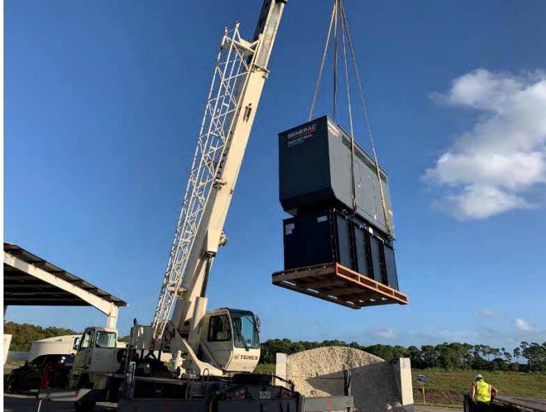
Offloading of Emergency Standby Generator Unit
