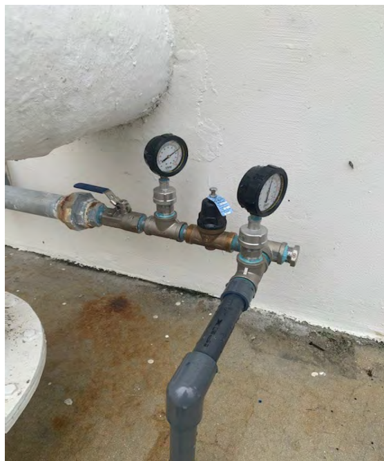
Headworks Odor Control - Service Water Pressure Reducer Assembly
