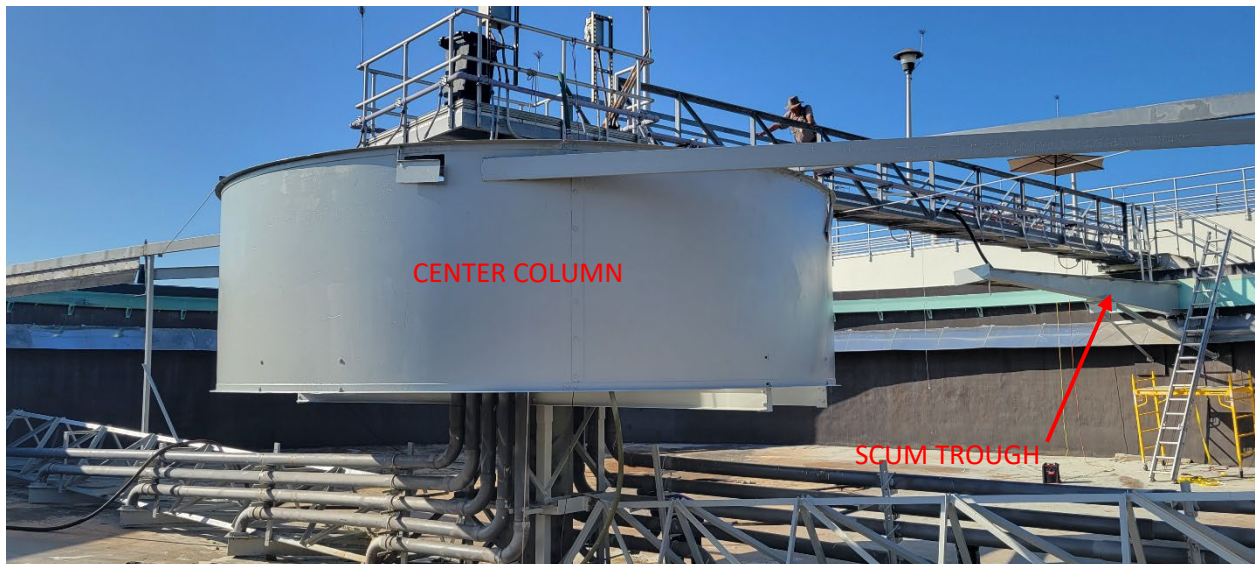
Clarifier No. 3 – Surface Preparation and Re-Painting of Center Column and Scum Trough
