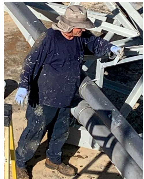
At left: Kemmm Peebles records confined space meter data on the confined space permit for entry to Clarifier 3. At right, Chris Whalen applies surface coating to the clarifier rake arm after days of blasting of corroded areas of the arm. Brian Davis performed the blasting activity.
