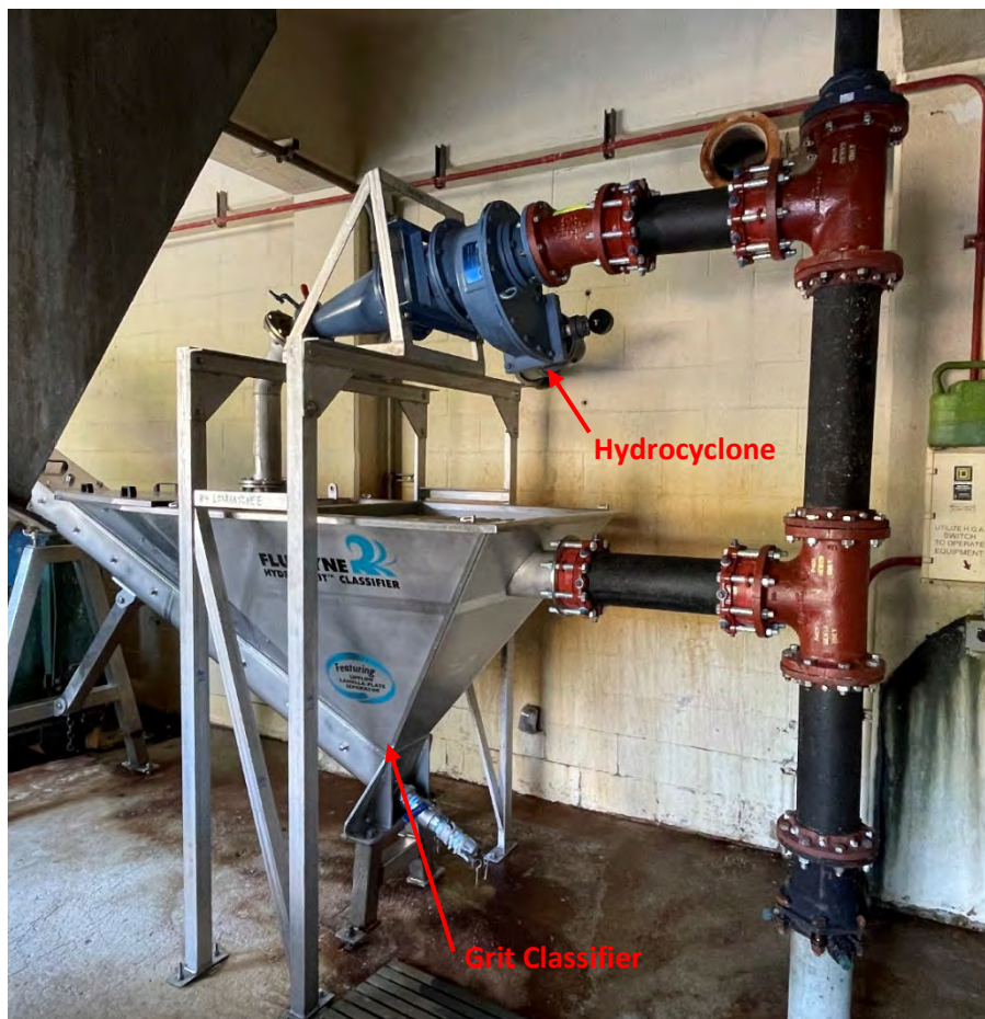
New Grit Classifier and Hydrocyclone Unit
