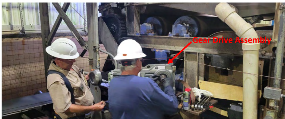
Replacement of Belt Filter Press Drive Assembly
