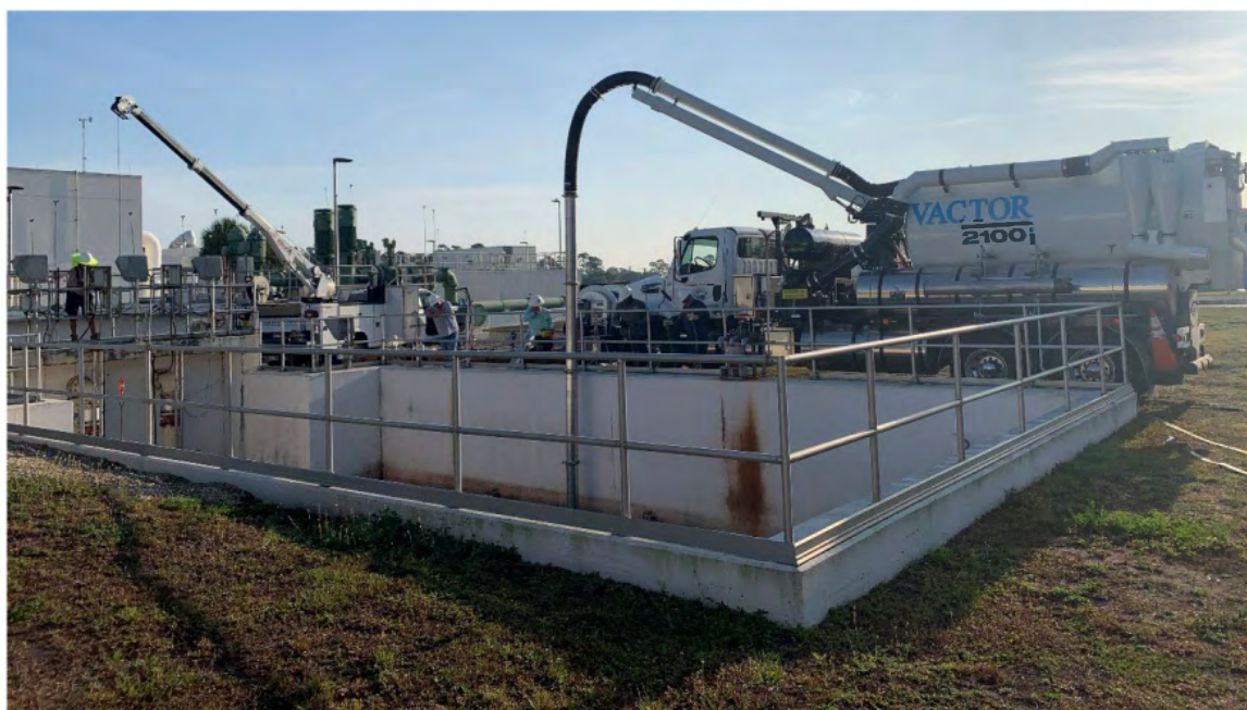
Annual Cleaning of Filter Backwash Waste Basin
