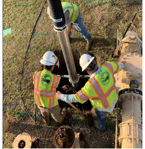
Construction Crew employees, Wyatt Fischbach and Tommy Cox utilize the Vac-Con's hydro-excavation and suction tube to evaluate the Influent Valve at the Raz Pit. Foreman Jason Broderick is directing the effort while Alex Smith (not shown) is remotely operating the vacuum tube.
