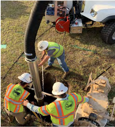
Construction Crew employees, Wyatt Fischbach and Tommy Cox utilize the Vac-Con's hydro-excavation and suction tube to evaluate the Influent Valve at the Raz Pit. Foreman Jason Broderick is directing the effort while Alex Smith (not shown) is remotely operating the vacuum tube.
