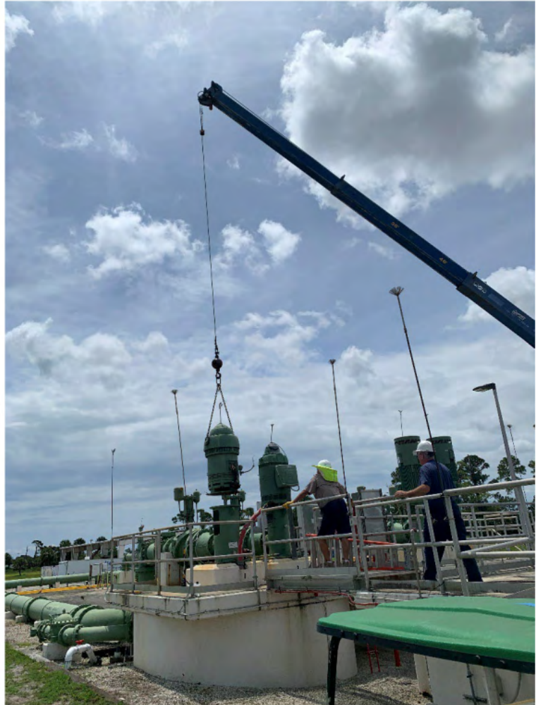
Maintenance Team Replacing IW Pump No. 1
