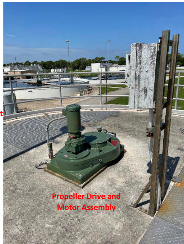
New Propeller Drive and Motor
