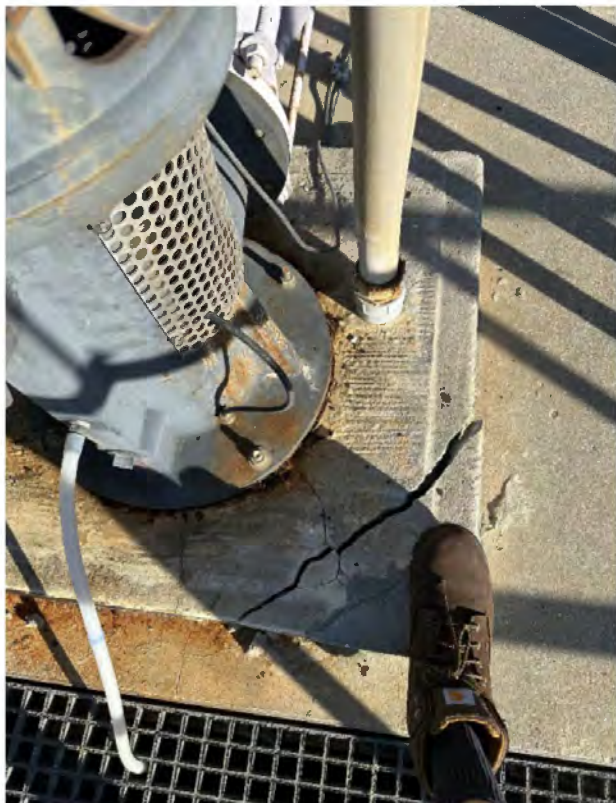
Broken/Cracked Concrete Pad at NPW Pump
