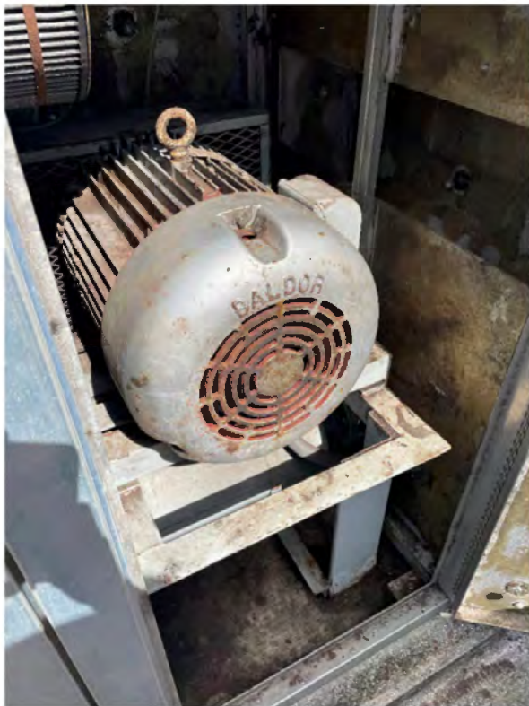
Sludge Storage Tank – Blower Motor
