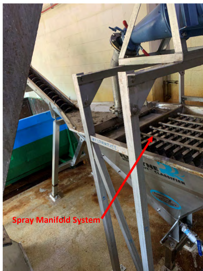
Grit Classifier Unit – Permanent Spray Manifold System
