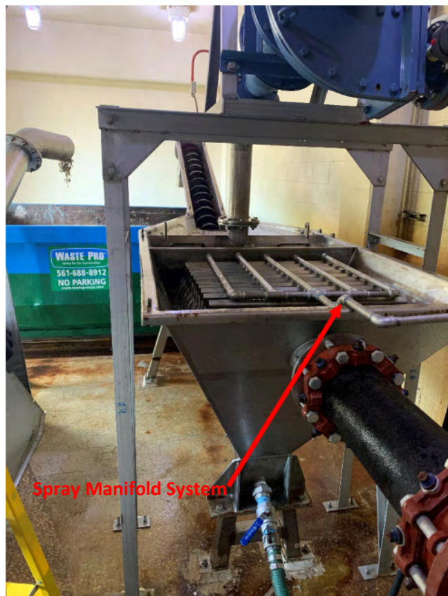
Grit Classifier Unit – Permanent Spray Manifold System
