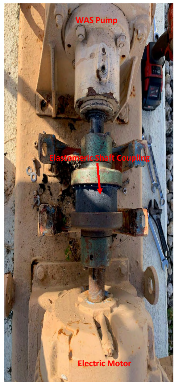
WAS Pump to Motor Shaft – Laser Alignment Procedure
