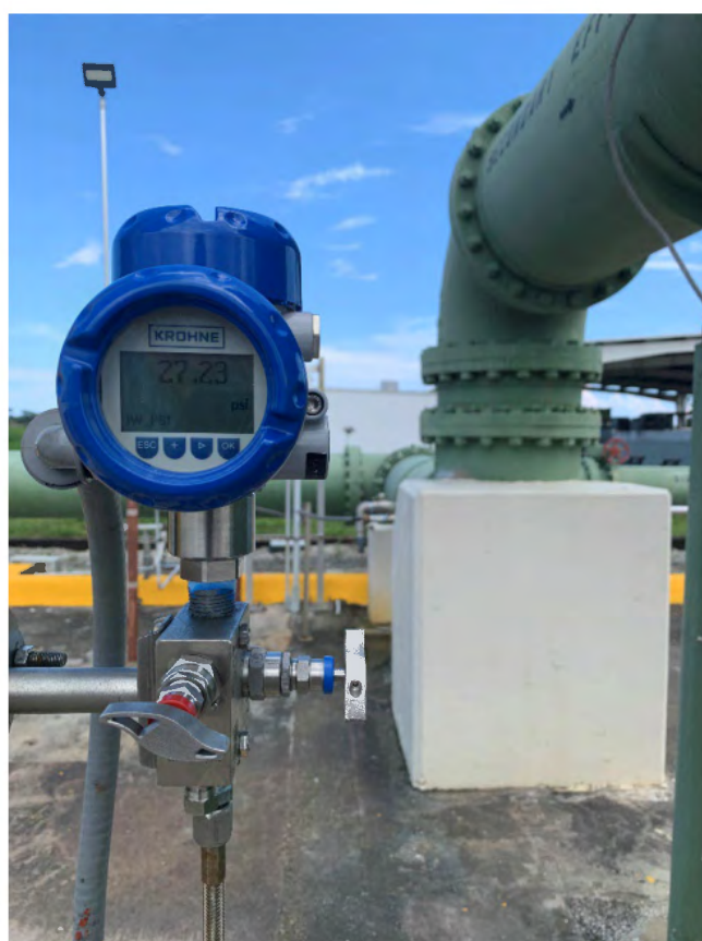
Deep Injection Well – Pressure Transmitter and SCADA Display
