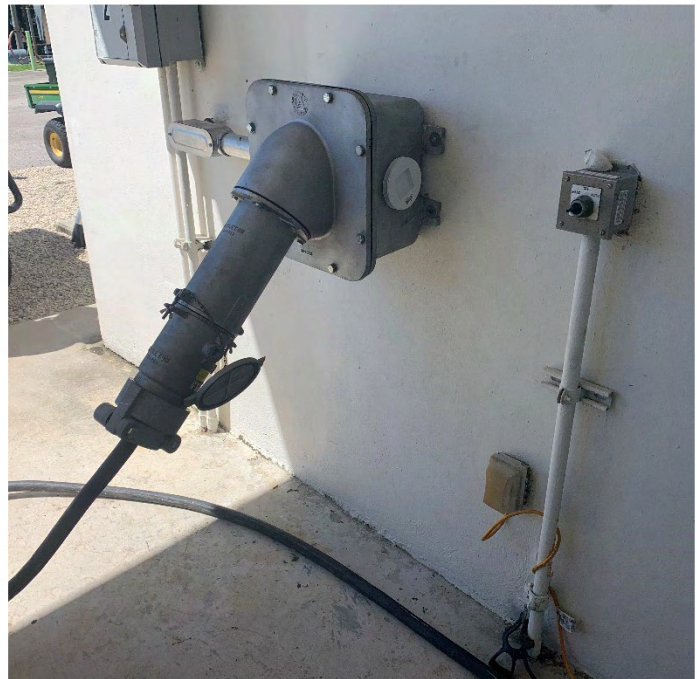
Installation of New 400A Towable Generator Plug at Headworks
